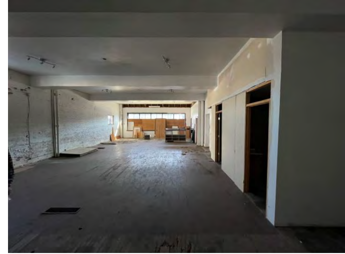
2 nd floor of building located on 348 Ellicott Street parcel.
