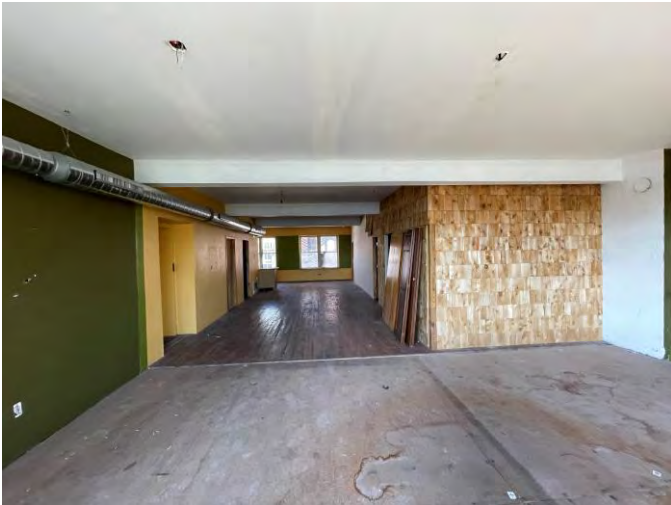
3 rd floor of building located on 348 Ellicott Street parcel.
