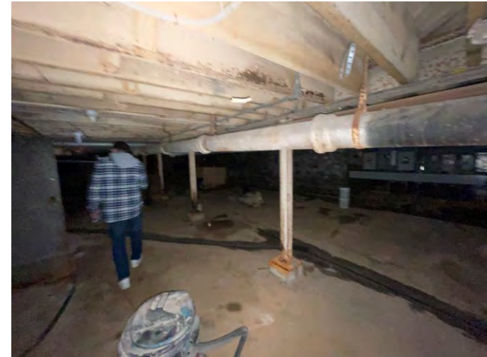
Basement of building located on 348 Ellicott Street parcel.
