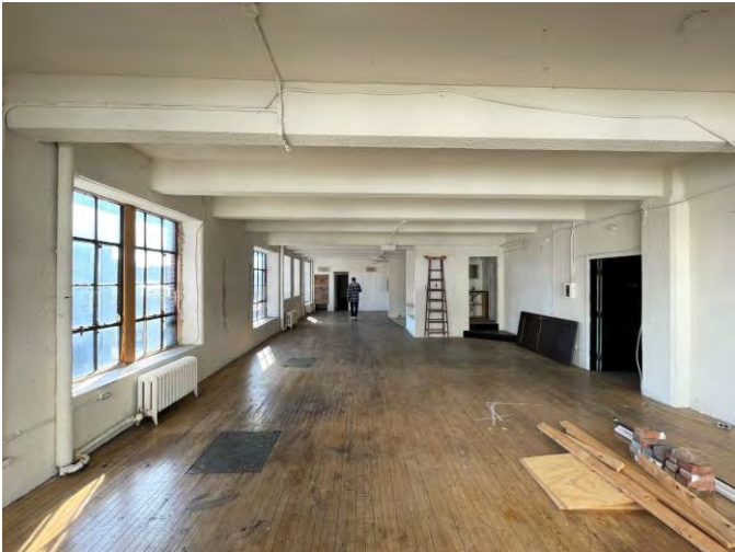
Inside building located on 23 East Huron Parcel. Facing south
