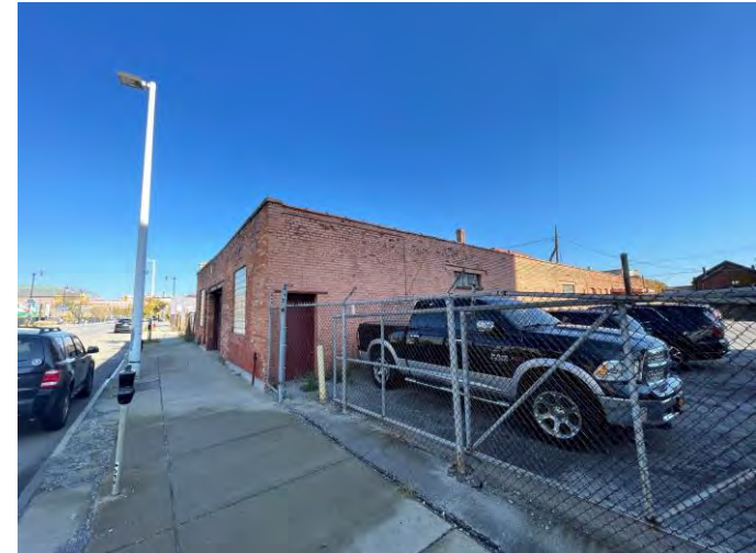
Building located on 379 Ellicott Street parcel. Facing northeast from Ellicott Street.
