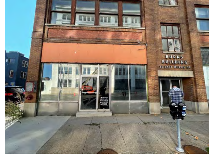
Building located on 23 East Huron Street. Facing south from East Huron Street.
