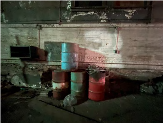
Drums located inside the building located on the 264 Oak Street parcel. Facing south
