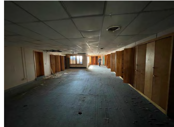
Inside building located on 23 East Huron Parcel. Facing north
