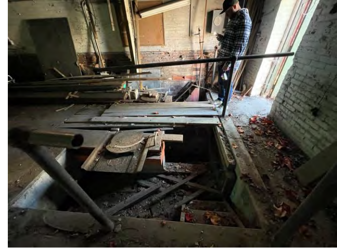
Broken floor bored and crawl space located inside the building located on the 264 Oak Street parcel. Facing south
