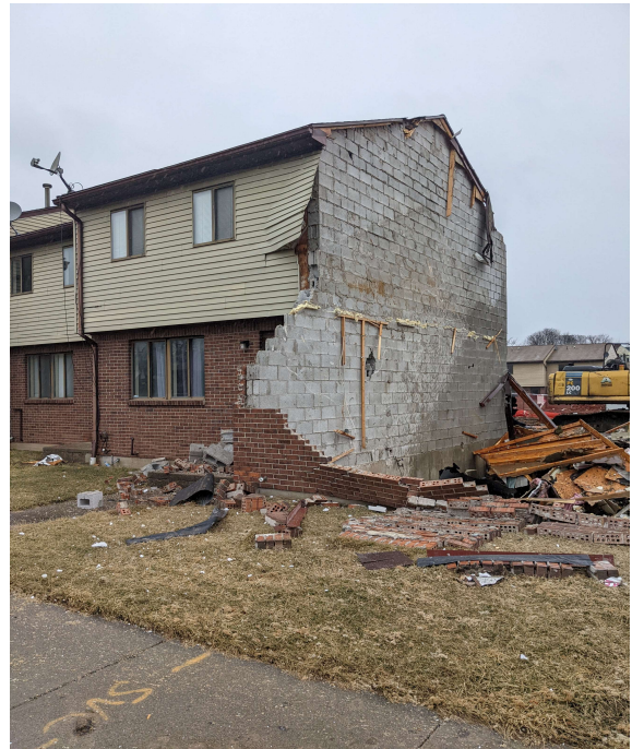
Demolishing Bldg. #53-58. Looking north.
