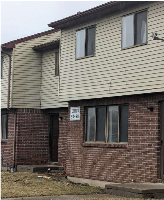
EBC prepping to demolish Bldg. #53-58.
