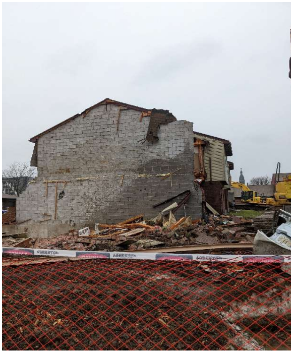
EBC prepping to demolish Bldg. #53-58. Looking south.
