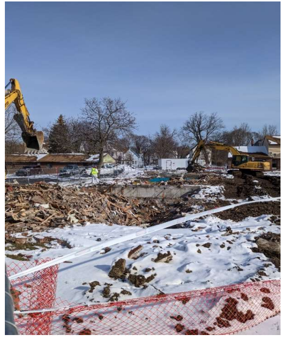
Bldg. #59-65 demo. Looking north.
