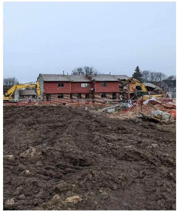
Bldg. #59-65 demo. Looking west.
