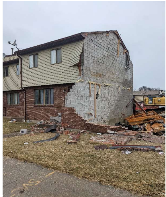
Demolishing Bldg. #53-58. Looking north.
