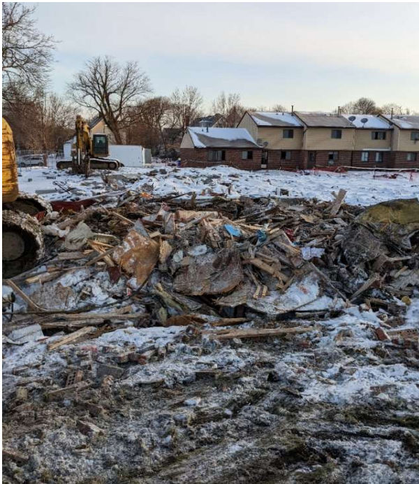
Bldg. #59-65 demo. Looking northwest.
