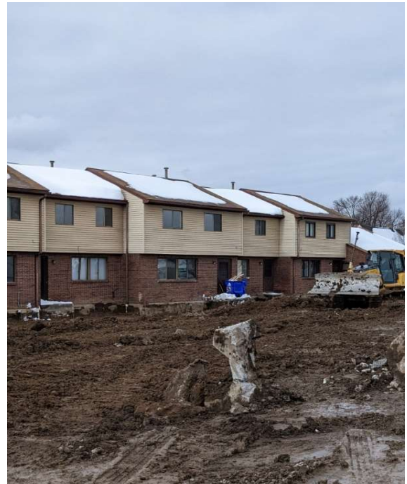
Bldg. #59-65, prepping to demolish. Looking south.
