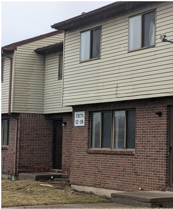
EBC prepping to demolish Bldg. #53-58.
