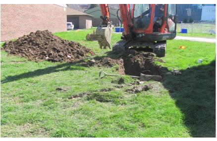
42. BH-22 location, excavator digging to broken pipe
