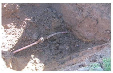
44. BH-22 location, broken copper pipe exposed
