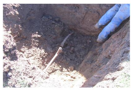
43. BH-22 location, broken copper pipe exposed
