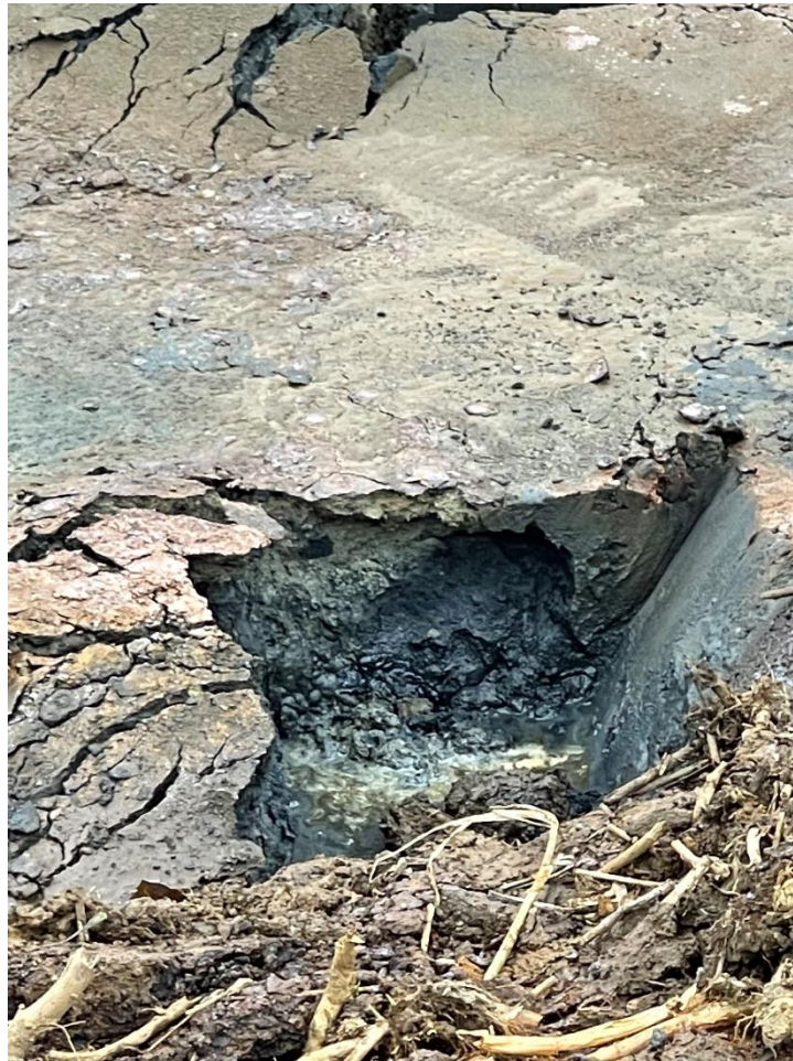
Photograph No. 3 Initial Investigation of Subsurface at Former ST24 Location May 26, 2022
