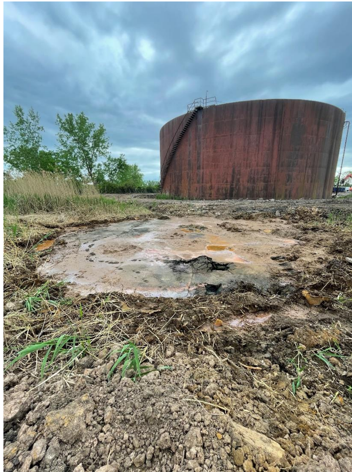
Photograph No. 2 Former Location of ST24 After Removal of the Base May 26, 2022
