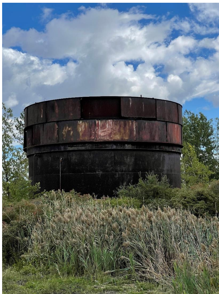
Photograph No. 1 ST24 Pentane Tank Before Demolition September 9, 2021
