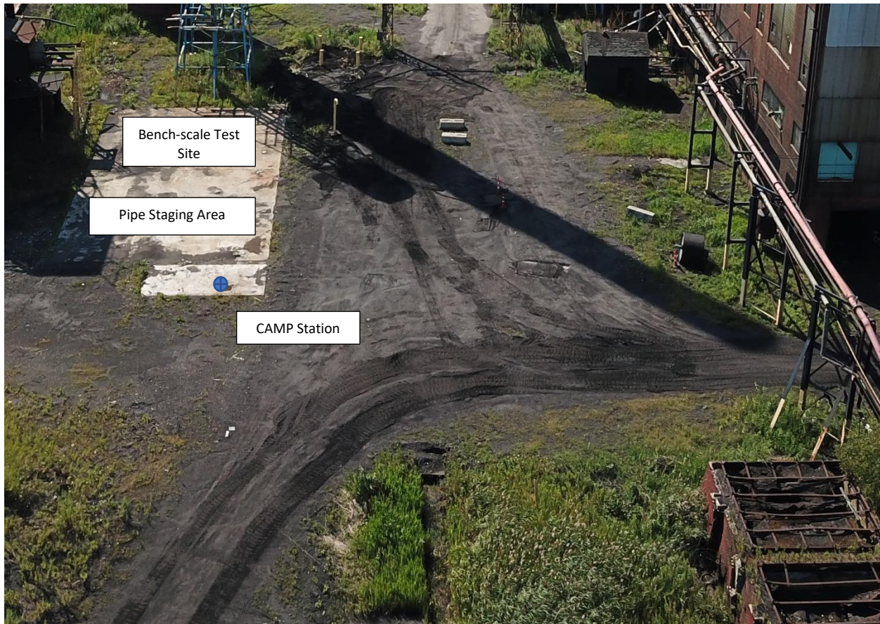
Photograph No. 2 Former Bag House Slab – Test Site
