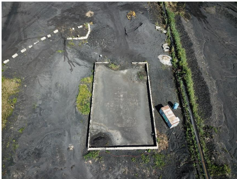
Mixing Pad, August 13, 2020 View Looking Down and Toward the East
