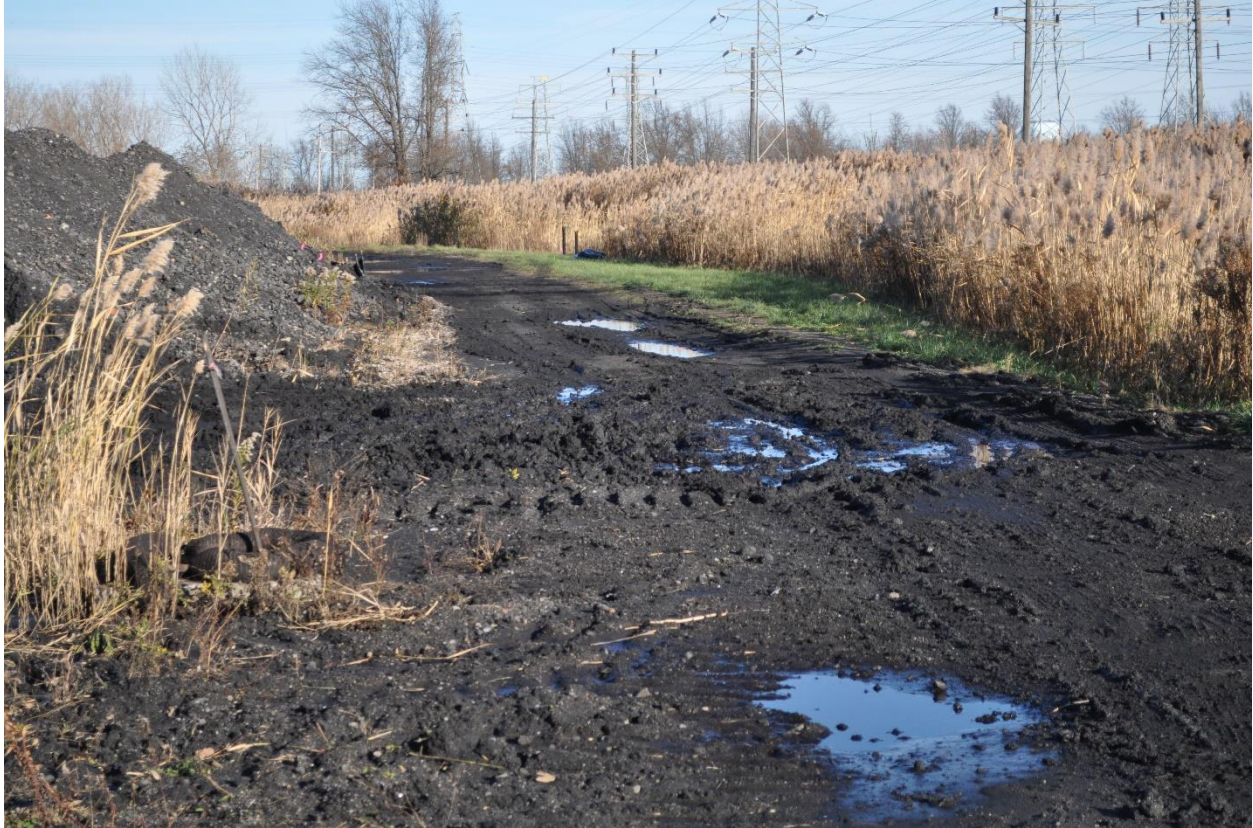
Photograph No. 7 South Ditch Road East of Curve TCC Road was Completely Degraded
