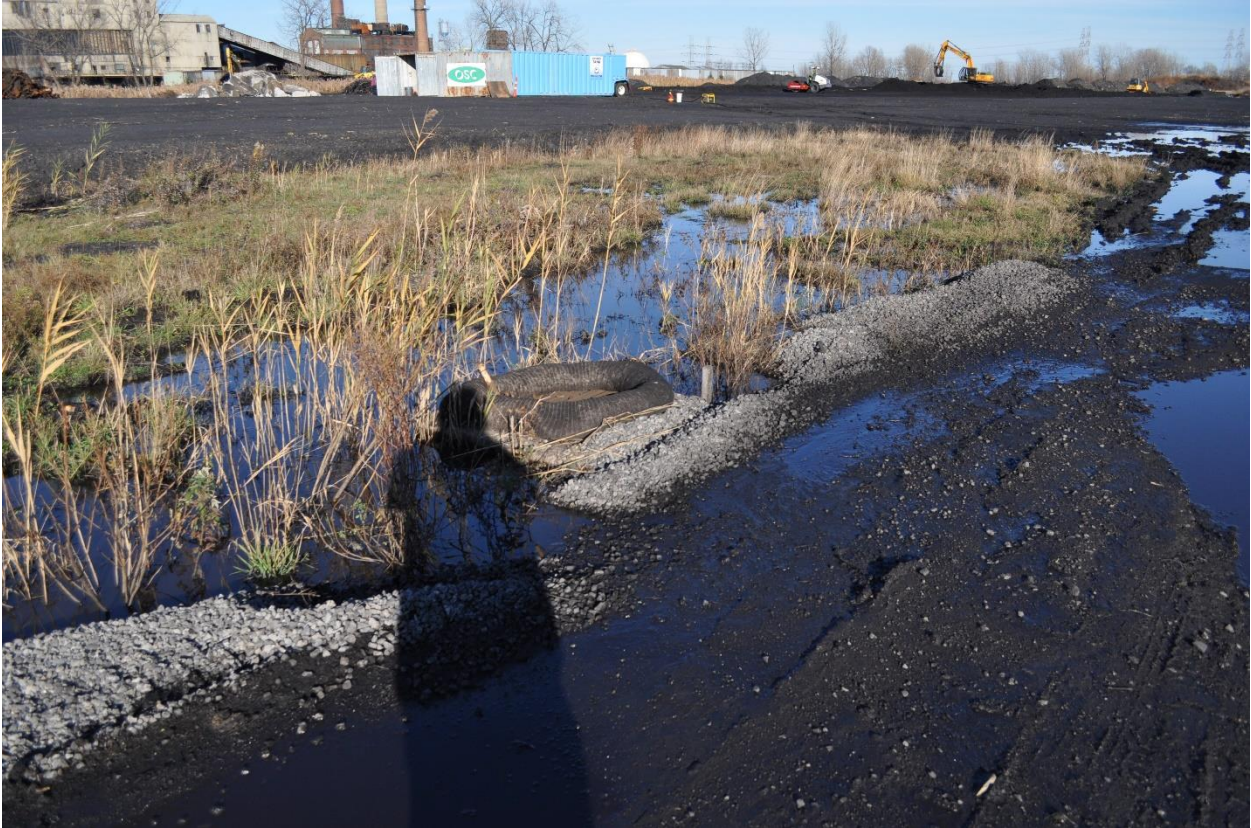
Photograph No. 2 Catch Basin No. 3 Note: Gravel Check Dams
