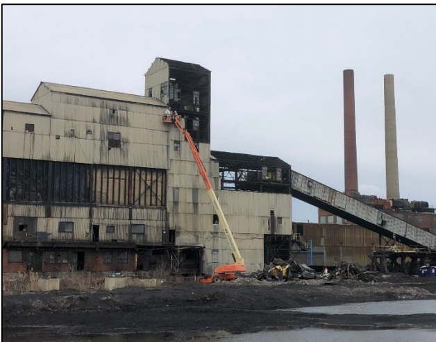
Asbestos panels being removed from the coal breaker building (March 2021).
