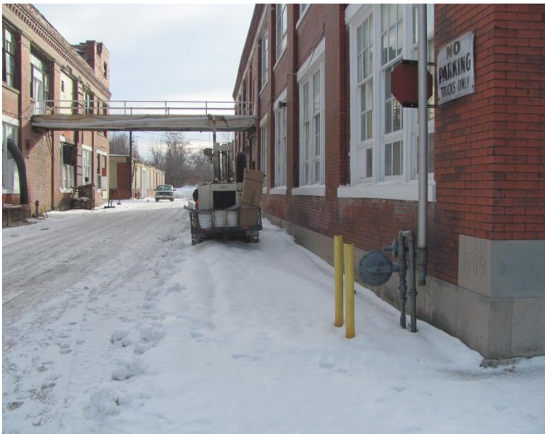
19. Location of BH-6 facing northwest
