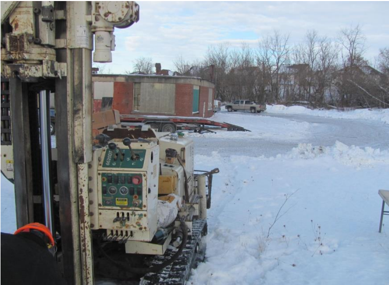
41. Location of BH-14 facing east at southwest corner of building 4
