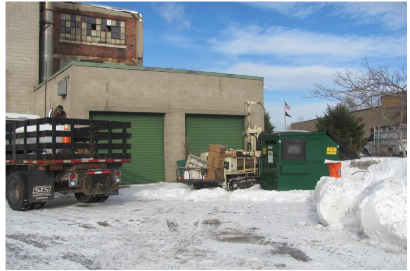
22. Location of BH-7 at southeast corner of Building 3
