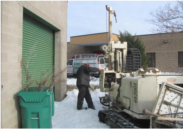
21. Location of Borehole BH-7 at southeast corner of Building 3
