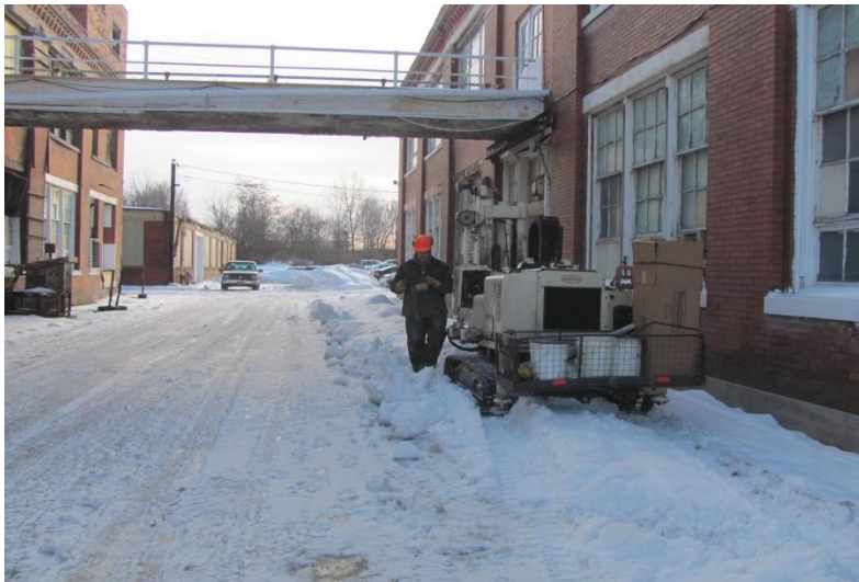
15. Location of BH-5 facing southeast
