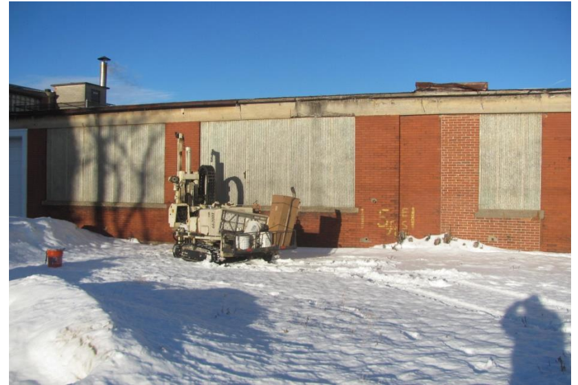
42. Location of Borehole BH-15 facing northeast adjacent to west side of Building 4
