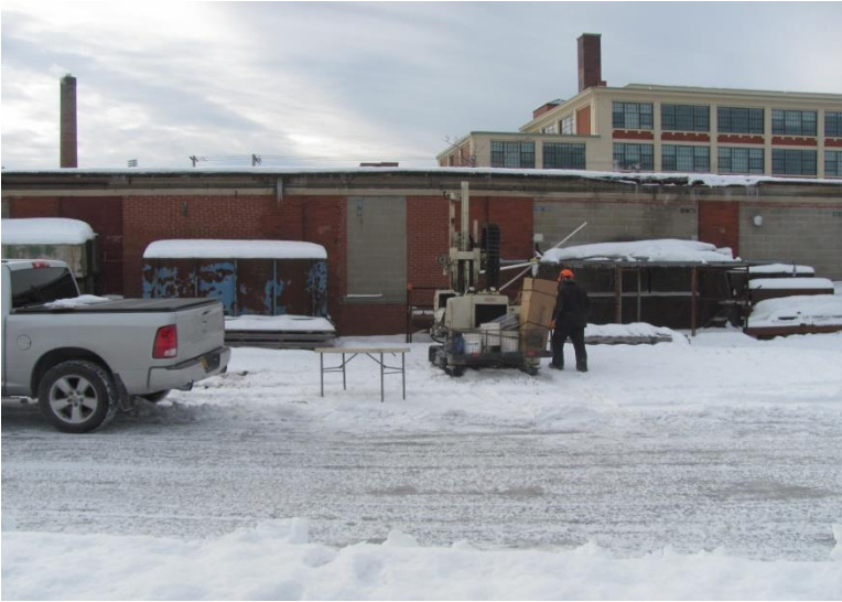
29. Location of Borehole BH-10 facing west-southwest at Building 4
