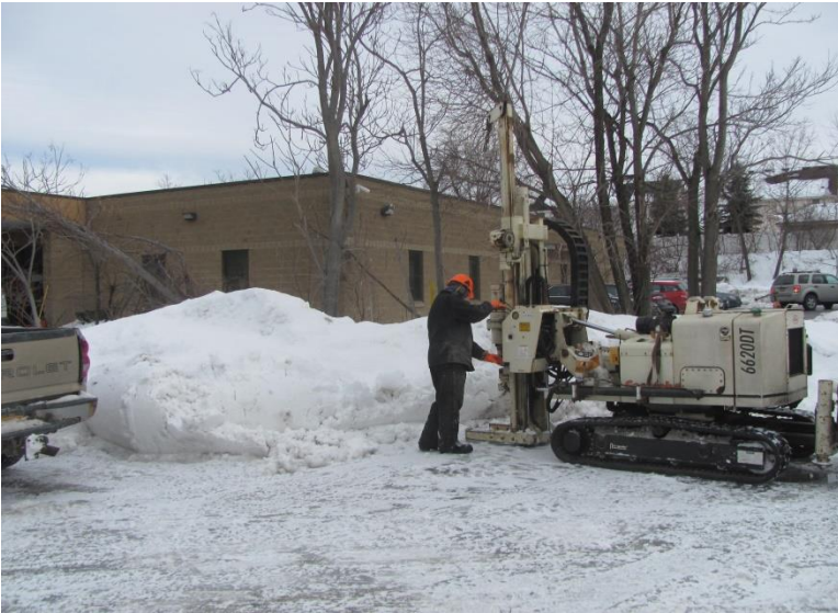
25. Location of BH-8 facing east
