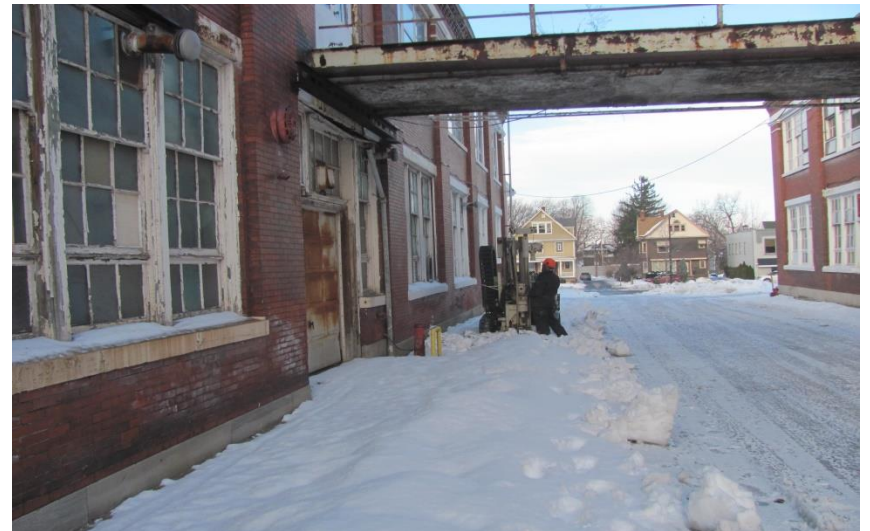
16. Location of BH-5 facing northwest
