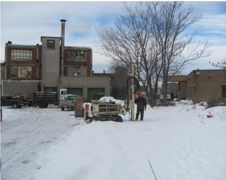
27. Location of BH-9 facing north-northwest at Building 3
