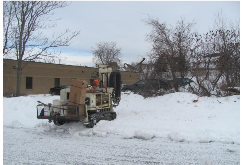
26. Location of Borehole BH-9 facing east
