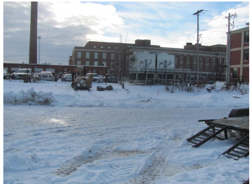
40. View of Borehole BH-14 facing west Bathune Lofts and Bennett High School
