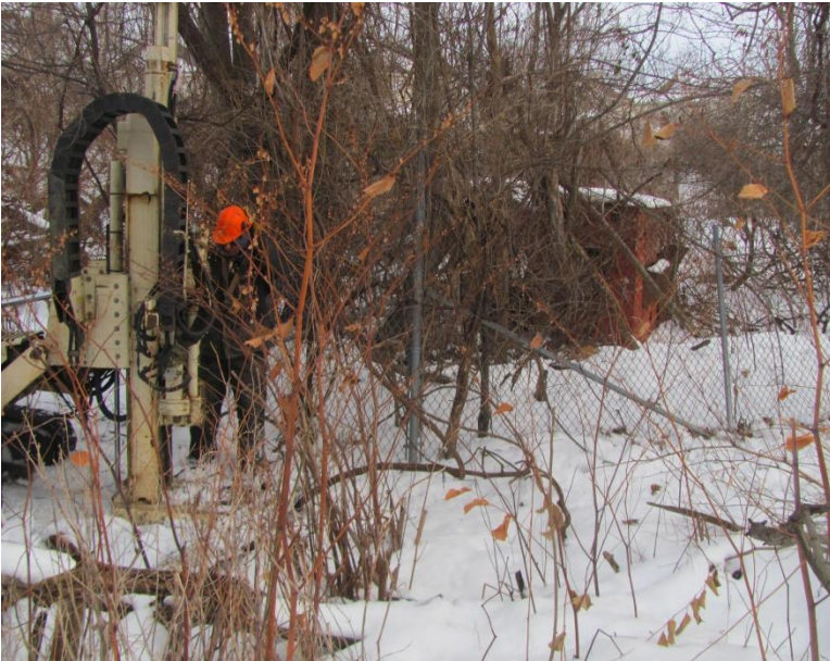
31. View of Borehole BH-11 location facing south at oil pump house
