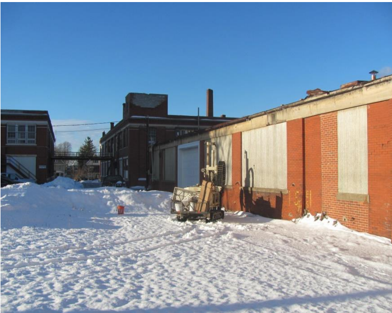
43. Location of BH-15 facing north-northwest
