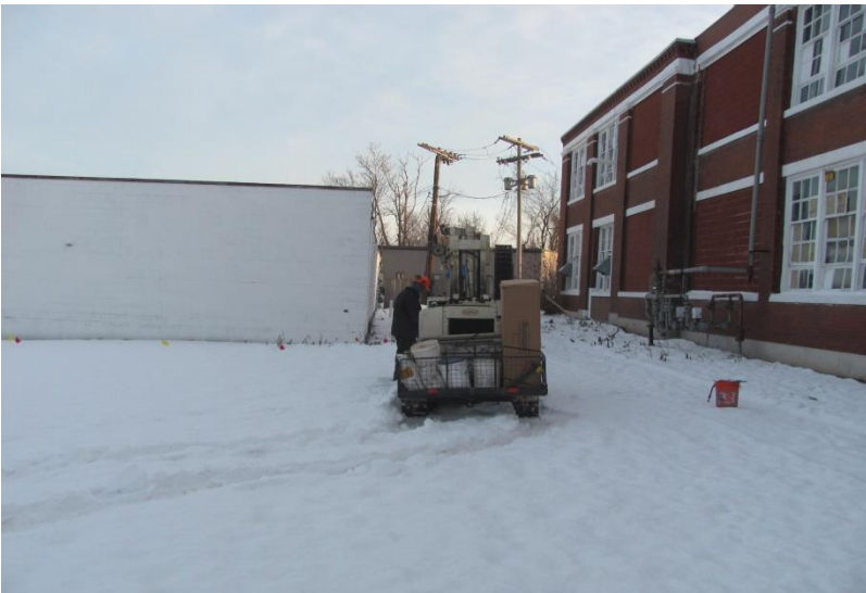
3. Location of BH-1 facing northeast
