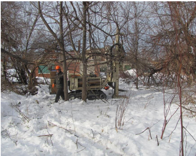
35. View of BH-12 facing north
