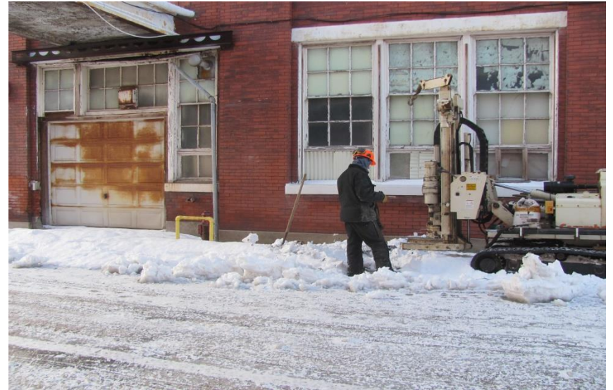
14. Location of Borehole BH-5 facing southwest and Building 2
