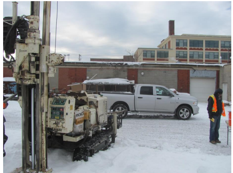
28. Location of BH-9 facing west at Building 4
