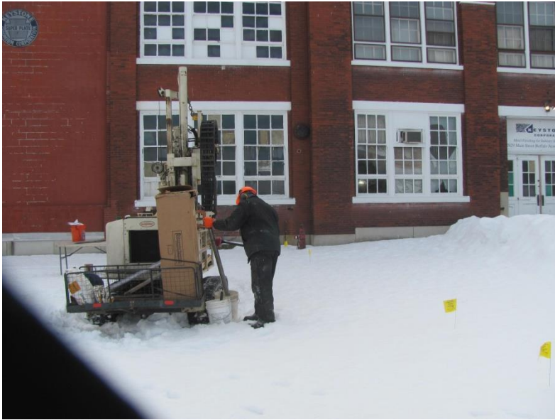
9. Location of BH-3 facing southeast at Building 3
