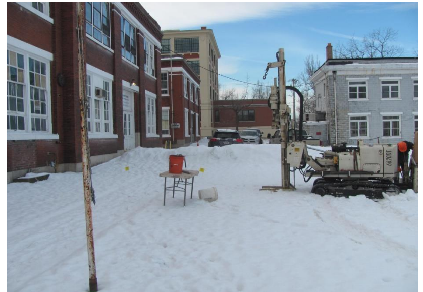
8. Location of Borehole BH-3 facing southwest
