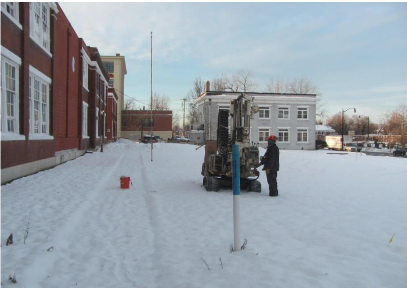
1. Location of Borehole 1 (BH-1) facing southwest along front of Building 3
