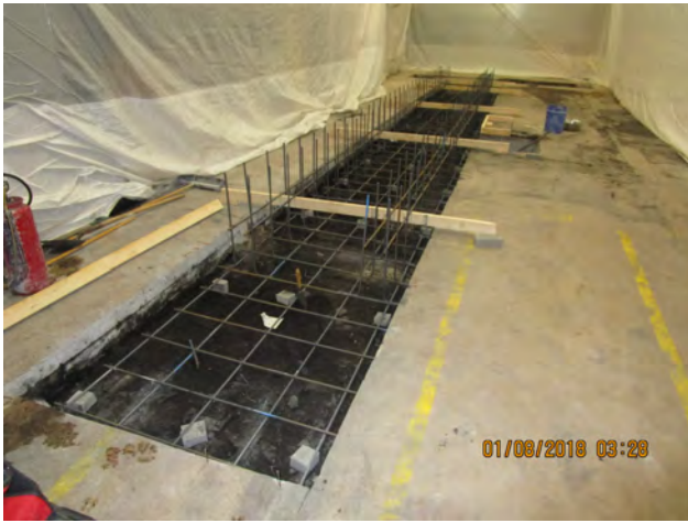
1. View of the Press Trench 01.
