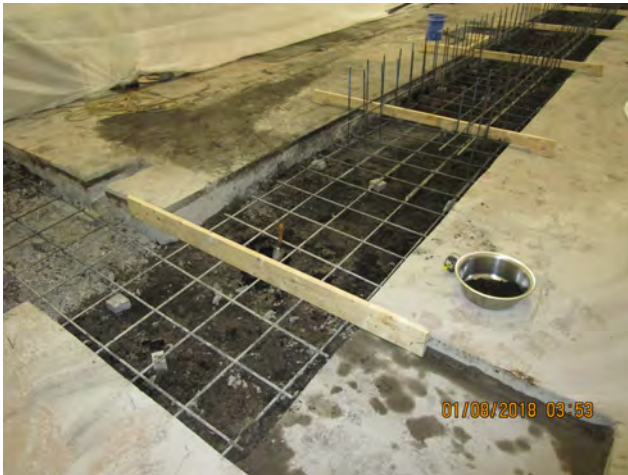
3. View of Press Trench 03.
