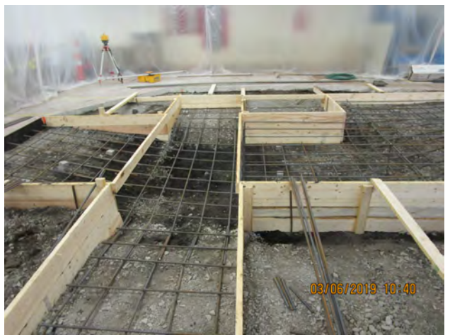
6. View of the Aerator Jogger Pit.
