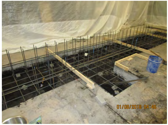
4. View of Press Trench 04.
