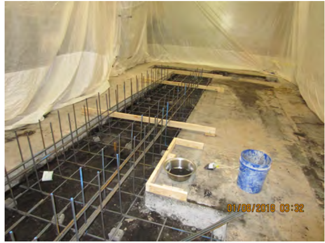
2. View of Press Trench 02.
