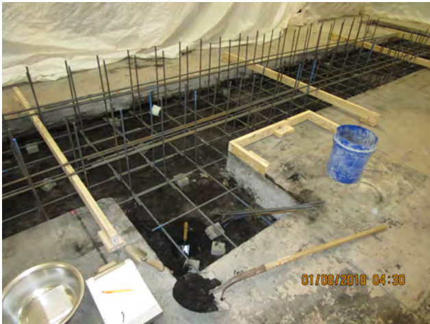
5. View of Press Trench 06.
