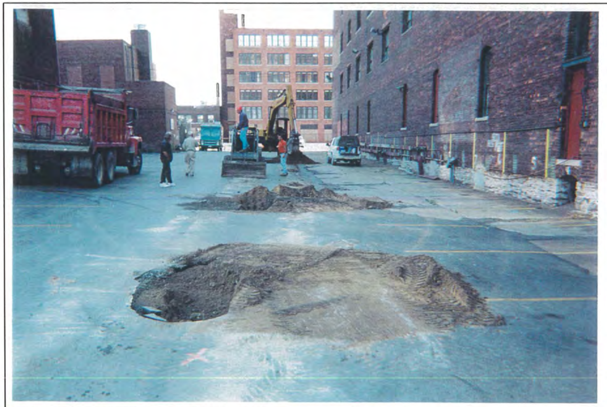
Photo 02: Test pits TP-2 (foreground), TP-3 and TP-4 locations and typical soil/fill lithology.
