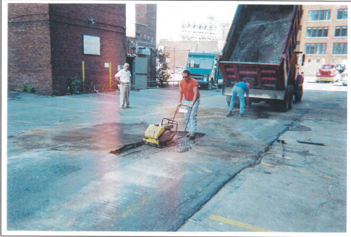
Photo 05: Test pit TP-5 showing typical select fill placement and compaction.
