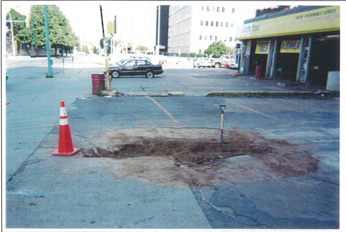
Photo 01: Test Pit TP-1 showing typical backfill of excavated material by NC.
