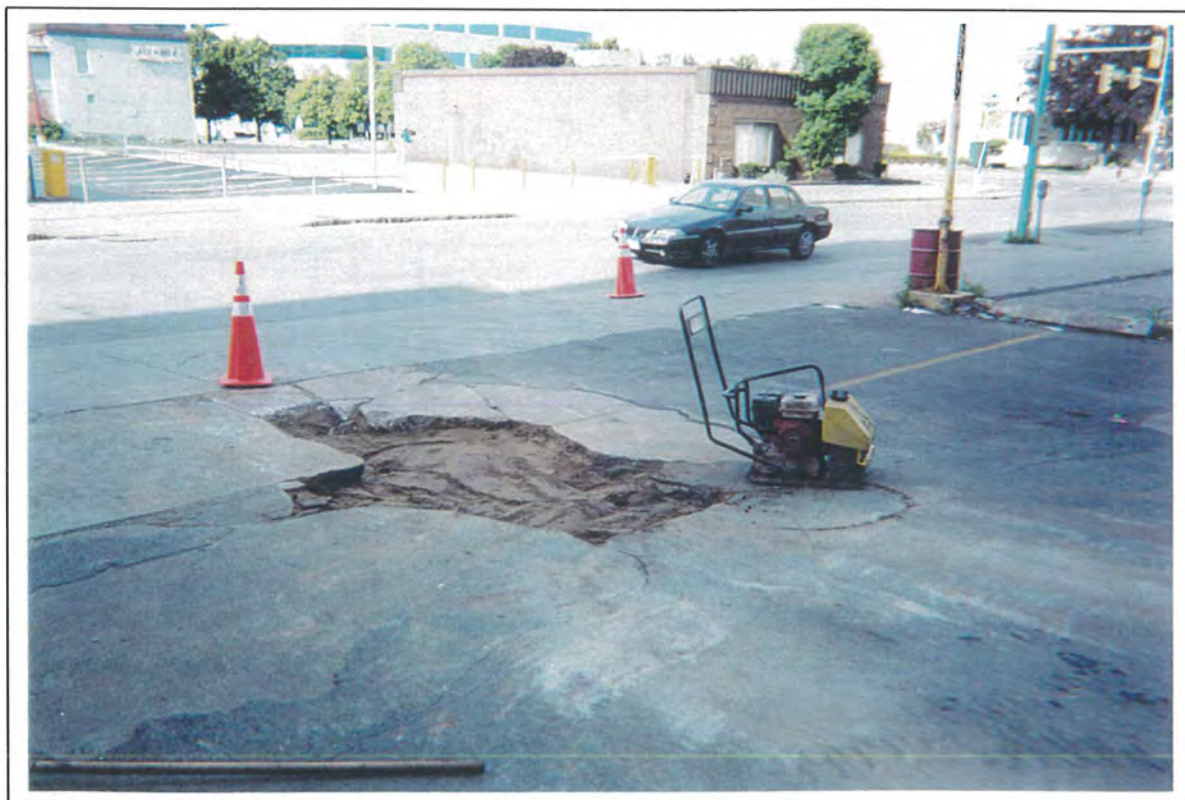
Photo 04: Test pit TP-1 showing typical backfill compaction with manual compactor.
