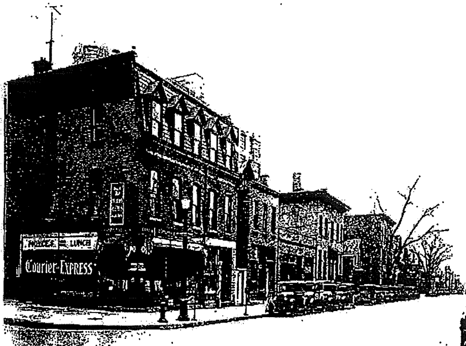
Goodell Street at Washington Street, looking east (ca. 1920). Note the Trico water tower on the upper left. (BECHS)
