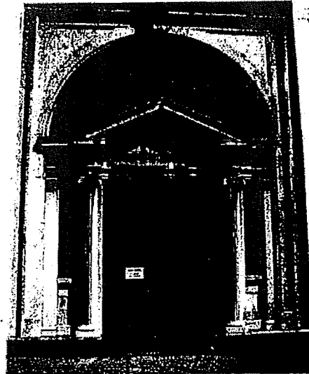
Detail of corner entrance (FAA)
