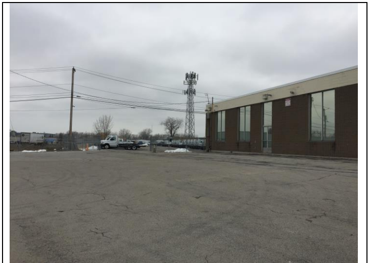
4. View facing west: Building, cell tower and western section
