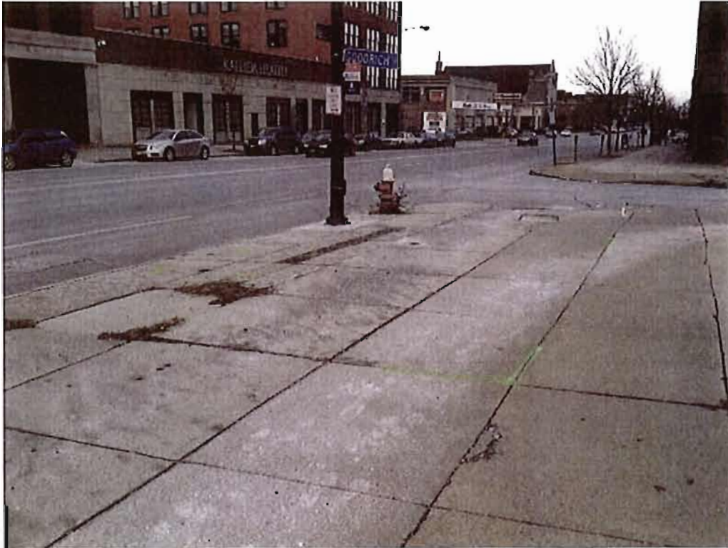
Photo #5: North Test Pit, View Facing Northwest (Green corners indicate safety fence boundaries.)
