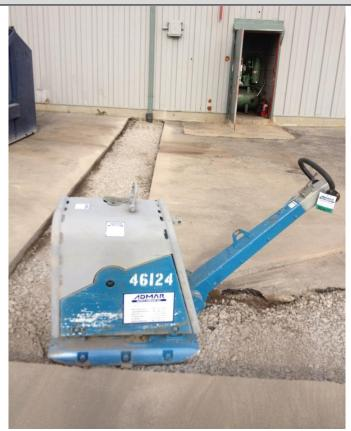
Crusher Run Compaction
