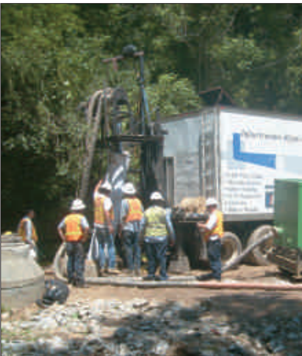
Easement installation of subdivision sewer rehab
