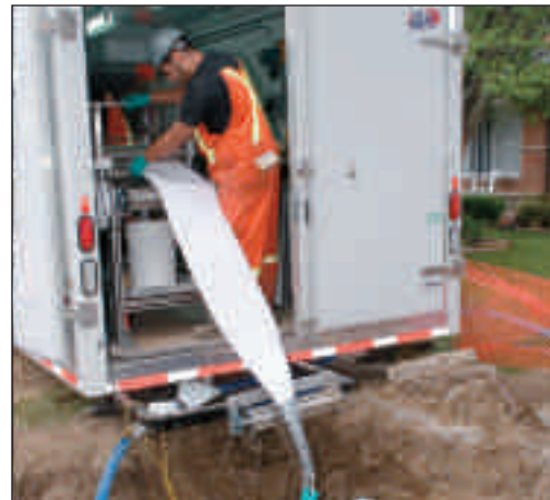
ASTM F1743 Pull & invert technology
