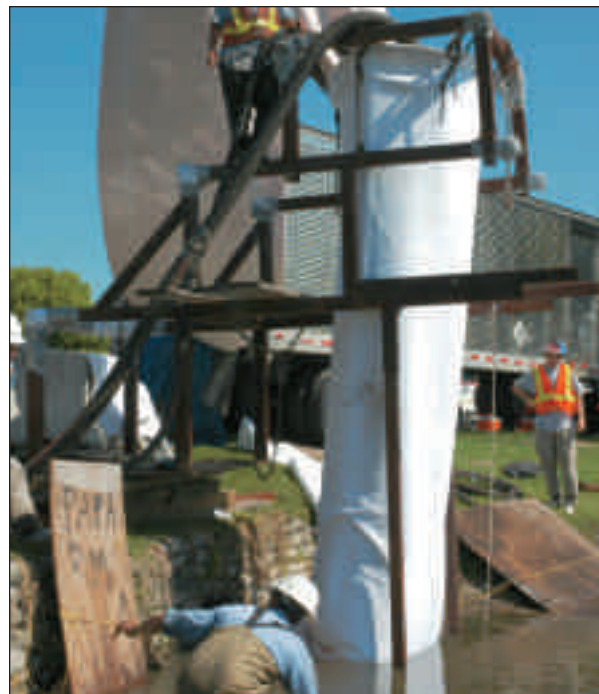
Subaqueous installation of CIPP into storm drain
