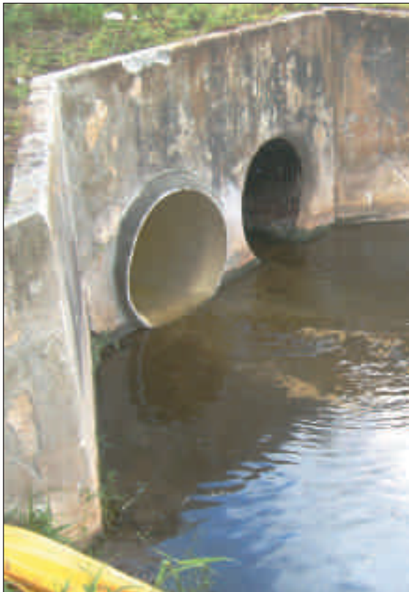
Trenchless renovation in storm drain application
