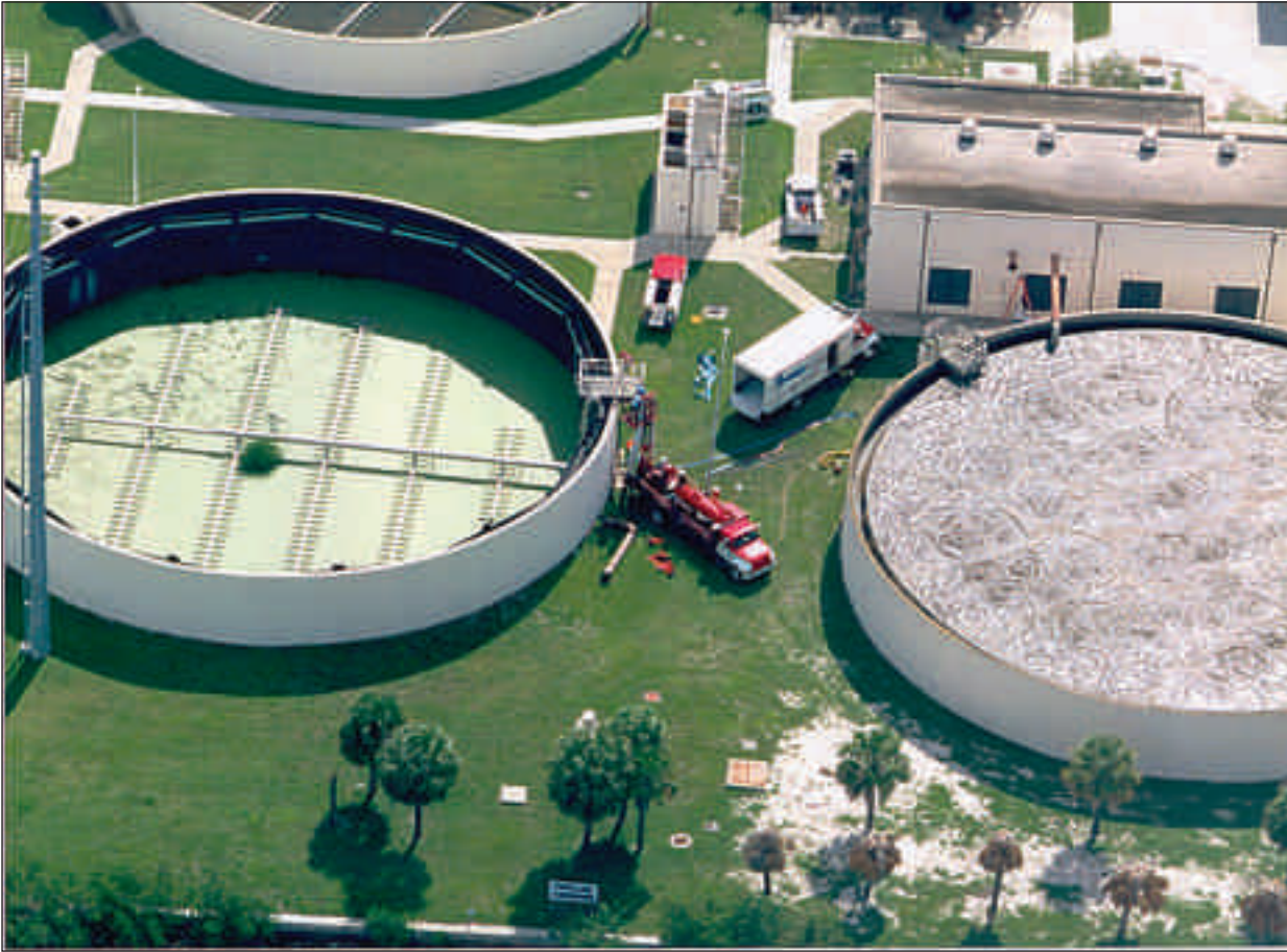
Clarifier pressure pipe rehabilitation at WWTP
