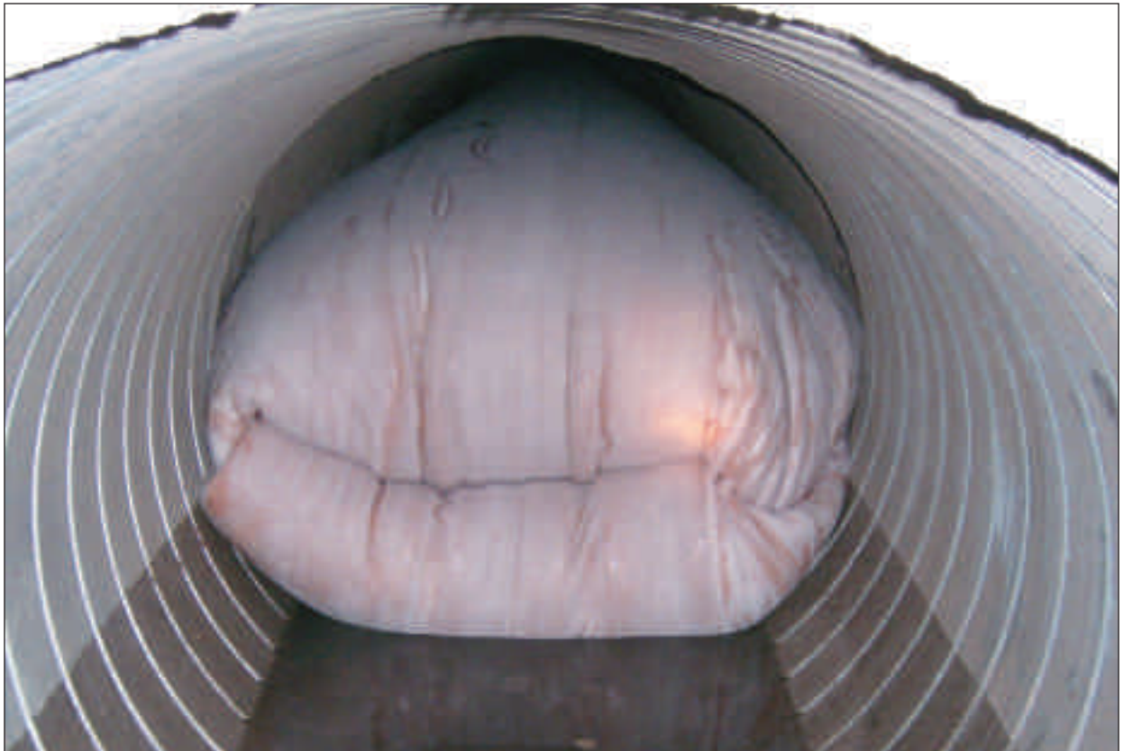
Frontal view of 60 inch diameter direct inversion
