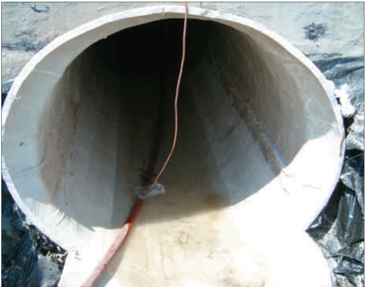
Finished outfall product at the headwall
