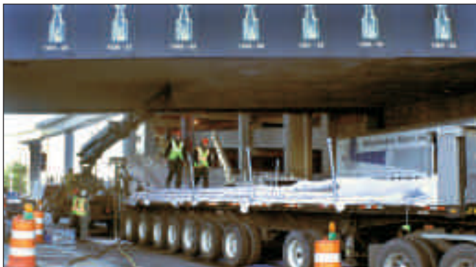
Large bore trenchless renovation in "tight quarters"
