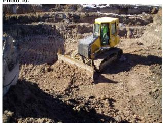
Photo 13: Excavation in progress (Looking North)
