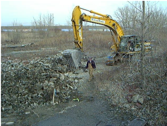
Figure 31 – TGA concrete demolition
