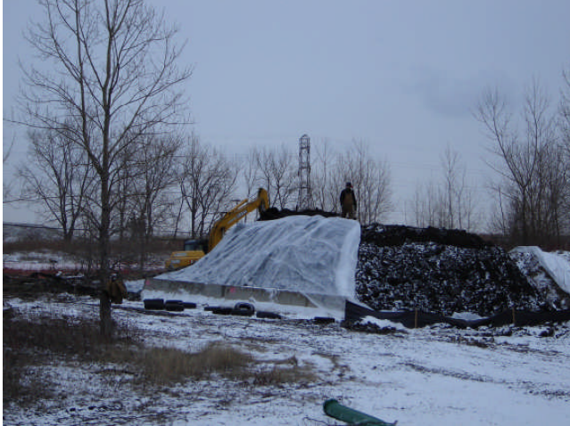
Figure 1: GC re -covering LNAPL spoil pile (facing south)
