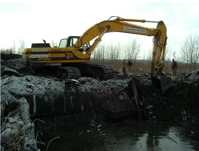
Figure 9 – LNAPL Excavation looking north-PM
