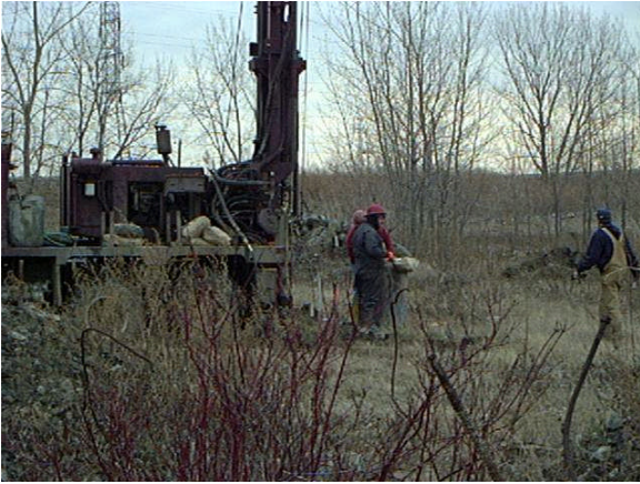
Figure 7 – MW removal 1
