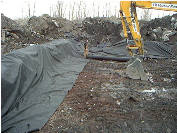
Figure 4 – Geofabric Install 1
