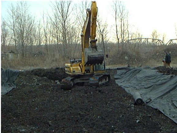
Figure 1 - Infiltration Basin prep 1
