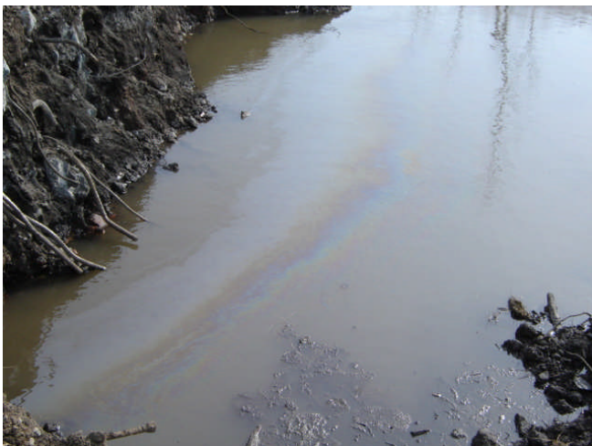
Figure DSC00015: Shows petroleum sheen on water in the LNAPL excavation (facing west)
