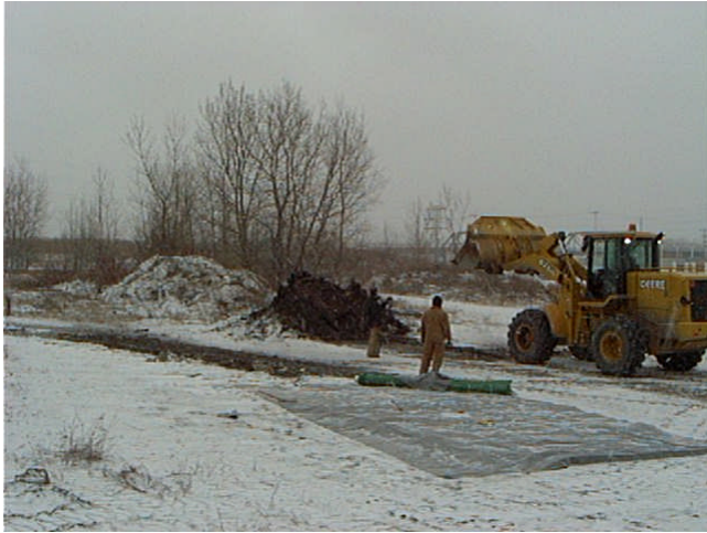
Figure 1 – LNAPL haul out road and DECON sand layer
