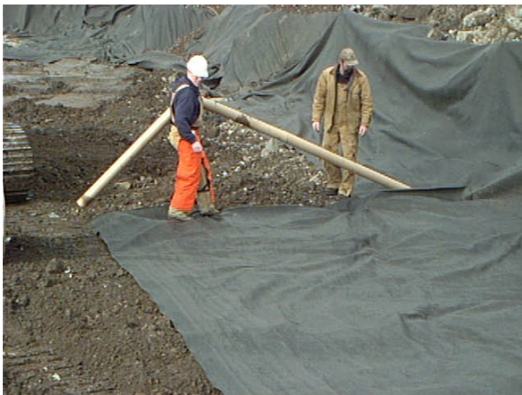
Figure 5 – Geofabric Install 2
