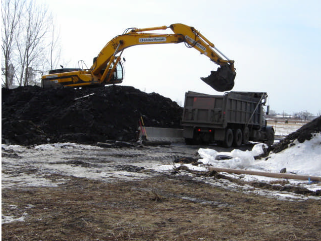
Figure DSC00016: GC loading out soil from the petroleum spill area, LNAPL stockpile (facing north)
