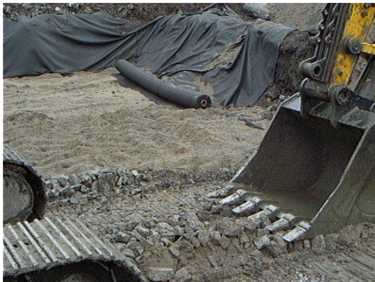
Figure 2 - Infiltration Basin Stone Layer 2
