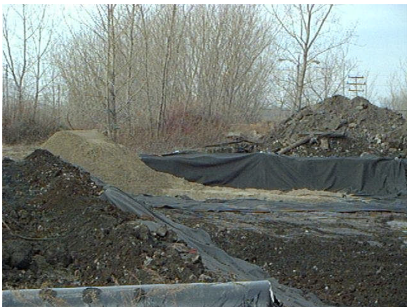
Figure 6 - Infiltration Basin-Sand Layer
