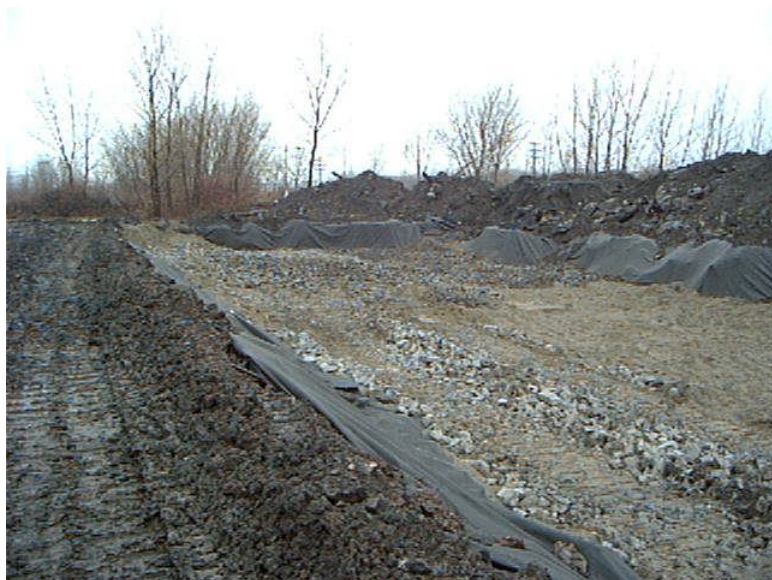
Figure 1 - Infiltration Basin Stone Layer 1
