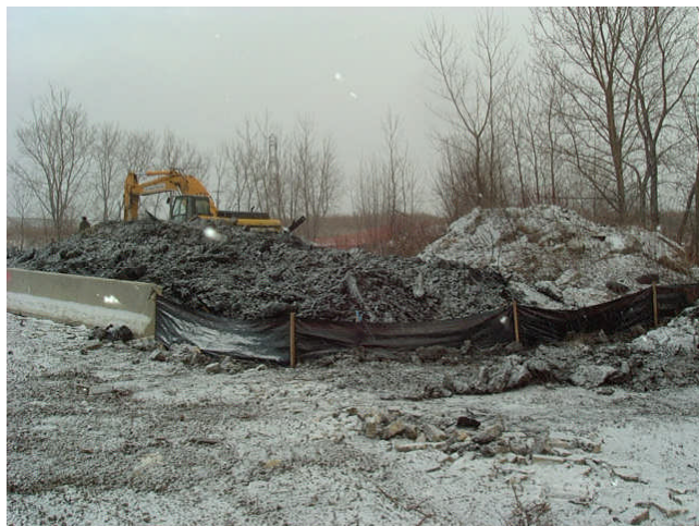
Figure 6 – Silt Fence at LNAPL Area-PM
