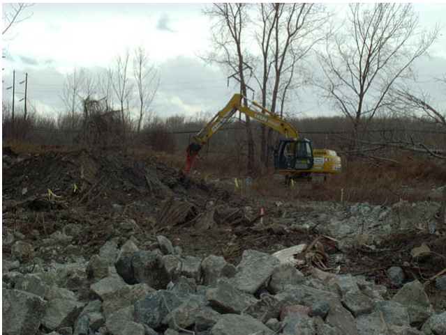
Figure 2 – Breaking concrete at the TGA-AM
