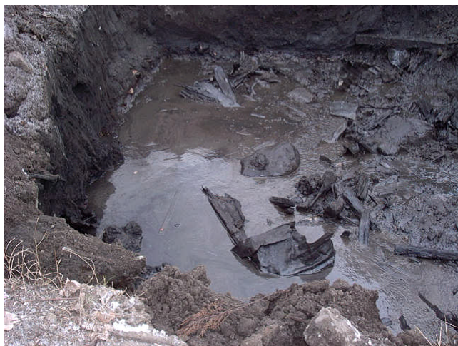
Figure 5 – LNAPL Excavation 11 AM
