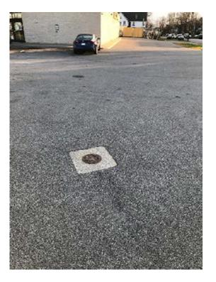
**Photo 4:** Existing groundwater monitoring well in northwestern portion of parking lot.
