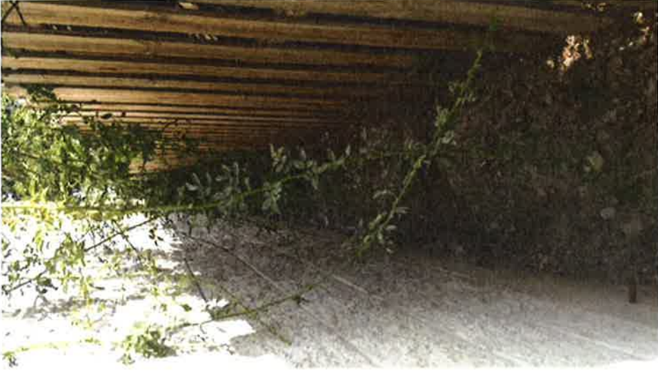
5. A view down the east side of the building.
