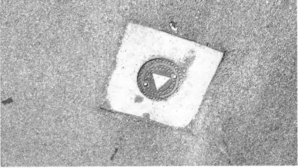
6. A standard monitoring well.
