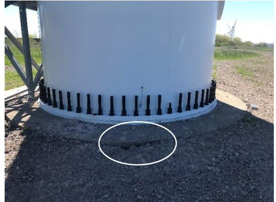
Closeup view of turbine foundation. Note location of inspection test pit.
