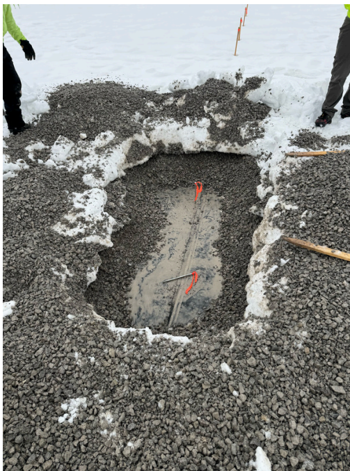
Photo 6 : Completed gravel removal
