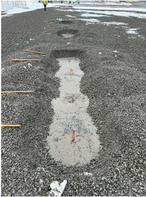
Photo 3 : Completed gravel removal
