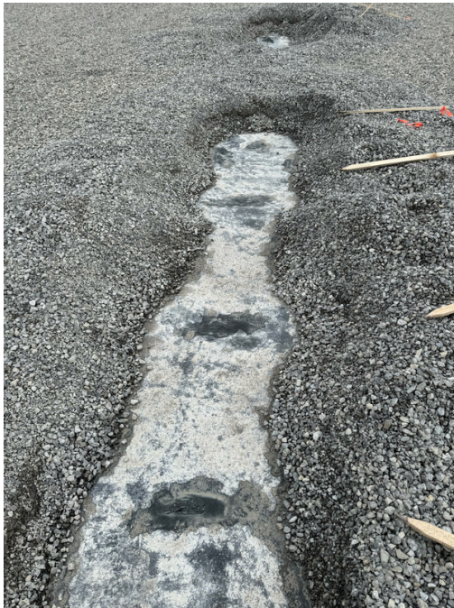
Photo 10 : Representative bead repairs
