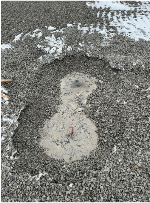
Photo 5 : Completed gravel removal
