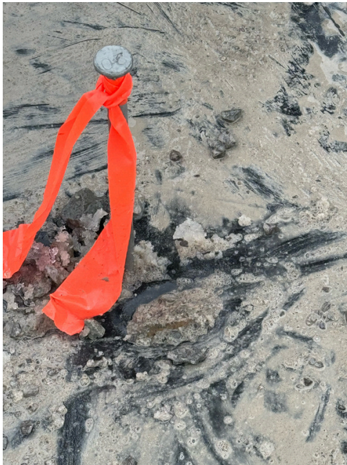
Photo 8 : Lath stuck in hole
