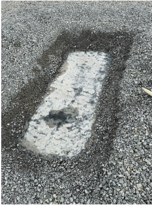
Photo 13 : Representative repair work
