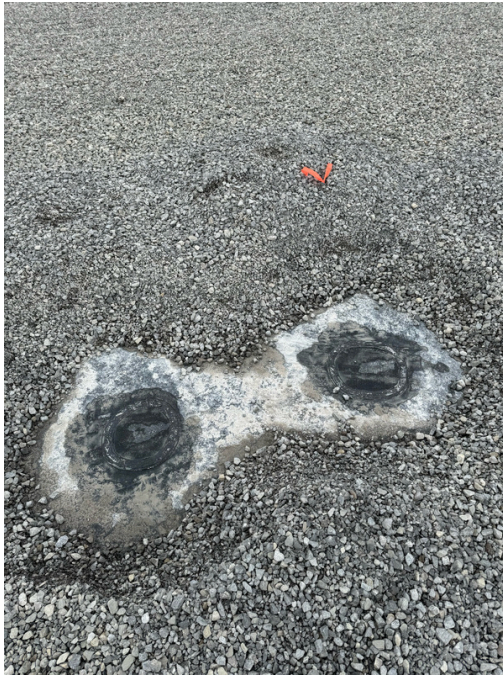
Photo 11 : Representative patch repairs
