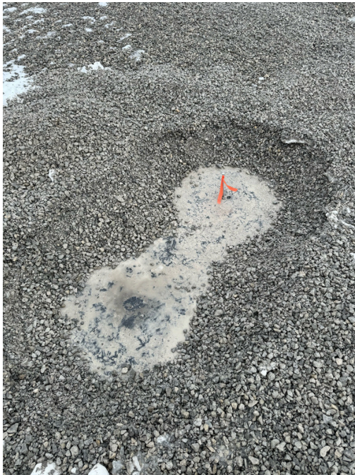
Photo 4 : Completed gravel removal
