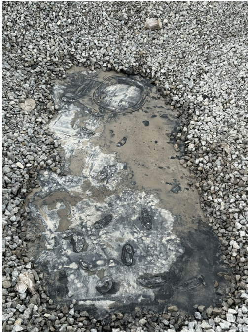
Photo 12 : Representative repair work
