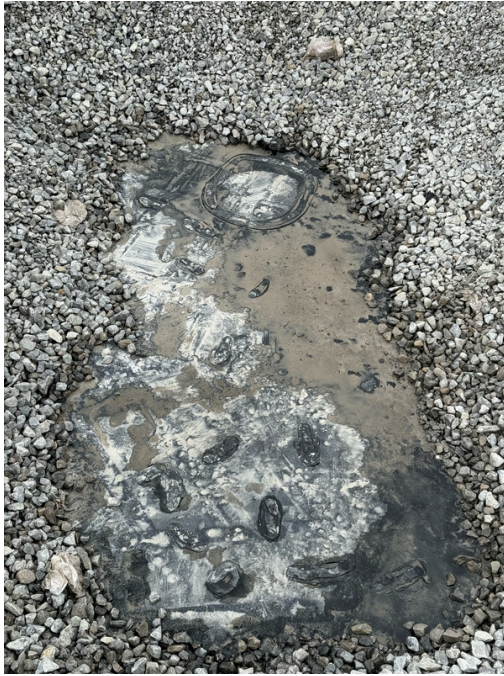
Photo 14 : Representative repair work
