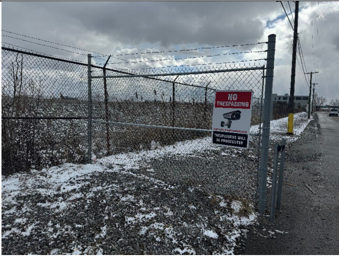
Completed Fence repair
