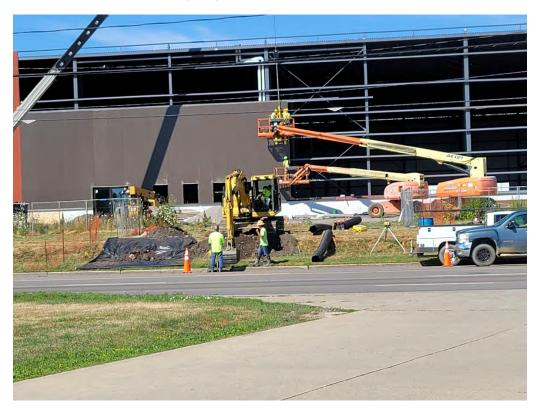
Photo 4-Excavation across Greenway trail for stormwater connector
