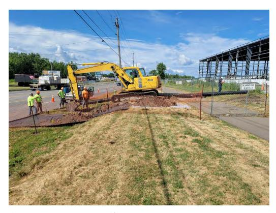
Photo 3-Excavation across Greenway trail for stormwater connector
