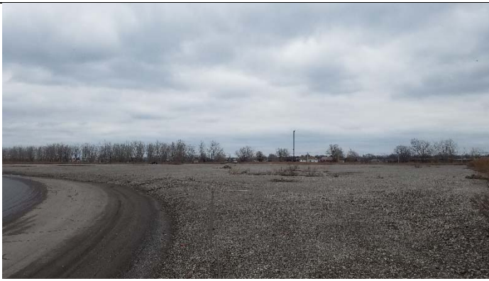
View of access road and cover from southwest corner facing north
