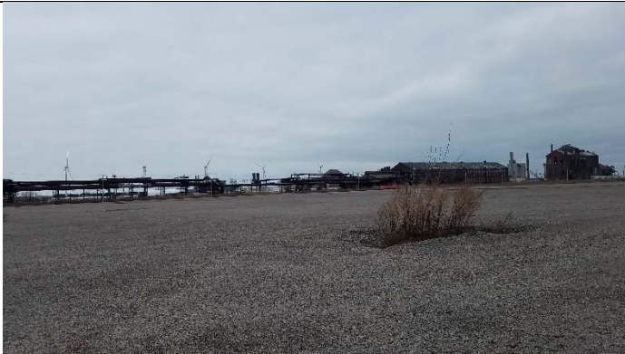
Site from southeast corner facing northwest
