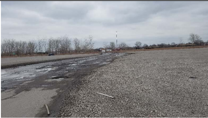
View of access road and cover from north boundary facing east
