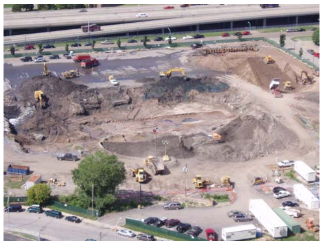
View of Excavation Activities August 2005
