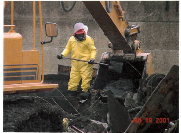
Residual material that couldn't be removed with equipment had to be shoveled out by hand.
