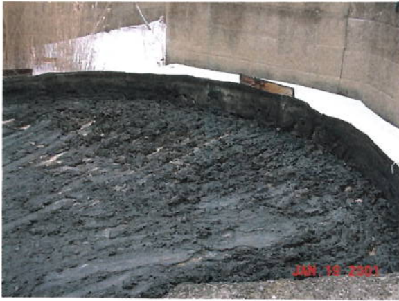
Residual material that couldn't be removed with equipment had to be shoveled out by hand.
