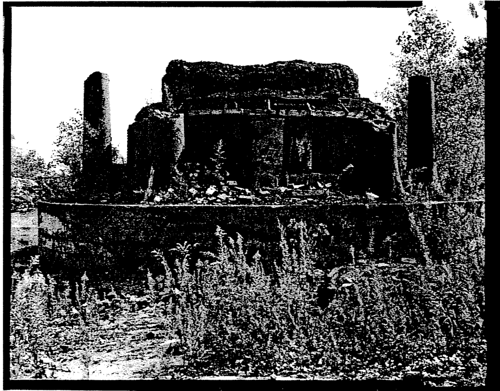
Photograph 4. West elevation of Hanna Furnace No. 3, facing east. Hanna Furnace Redevelopment Project, Buffalo, Erie County, New York (PCI 2001).
