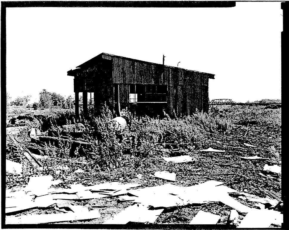
Photograph 12. North and west elevations of Hanna Furnace Filter House, facing east. Hanna Furnace Redevelopment Project, Buffalo, Erie County, New York (PCI 2001).
