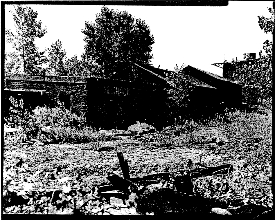
Photograph 9. South elevations of Hanna Furnace Oil Shack and Coal Storage Building, facing south. Hanna Furnace Redevelopment Project, Buffalo, Erie County, New York (PCI 2001).
