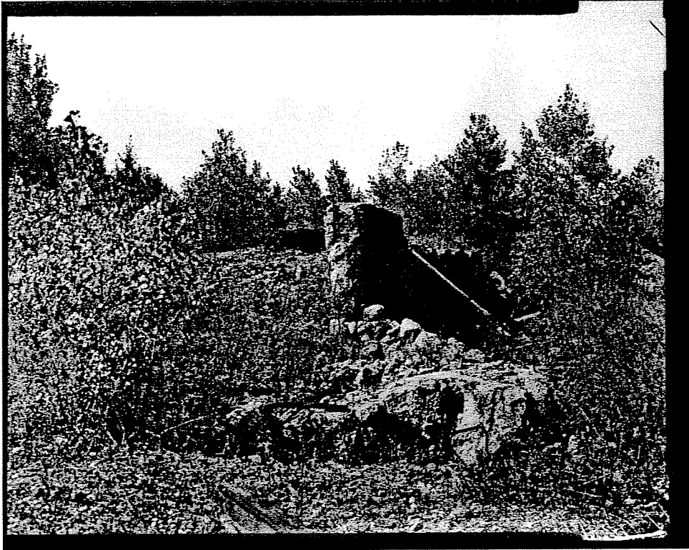
Photograph 6. Hanna Furnace No. 1 with slag dump and drain, facing southwest. Hanna Furnace Redevelopment Project, Buffalo, Erie County, New York (PCI 2001).
