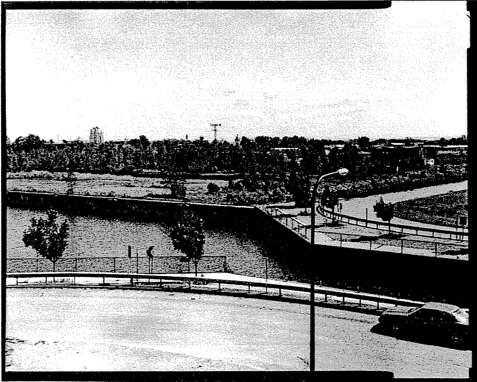
Photograph 14. Union Canal with Hanna Furnace complex in background from NY Route 5 Bridge, facing southeast. Hanna Furnace Redevelopment Project, Buffalo, Erie County, New York (PCI 2001).
