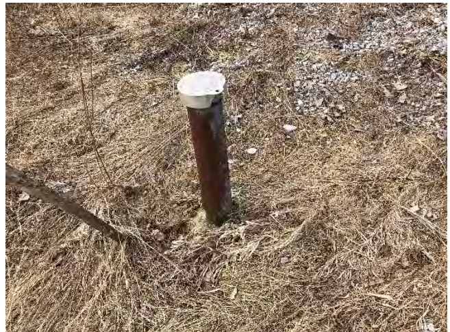
Photo No. 6 OW-9/MW-3 missing lock
