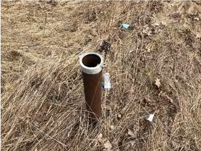
Photo No. 3 OW-5 missing cover & lock
