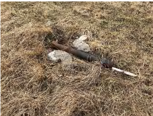
Photo No. 17 Unknown well destroyed
