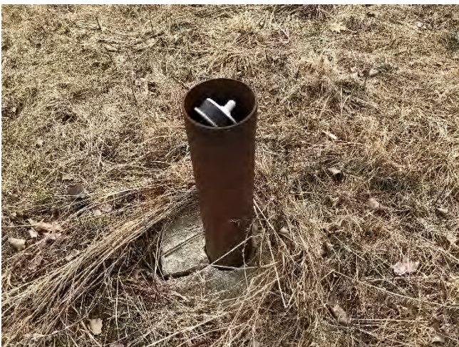
Photo No. 11 IW-11 cover broken off
