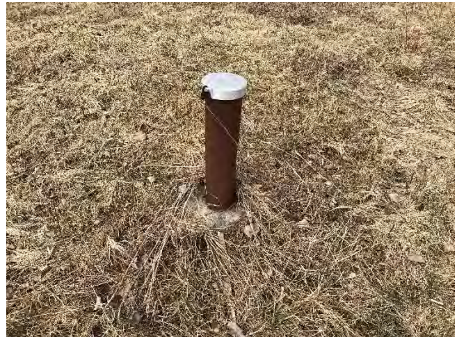
Photo No. 10 IW-10 in good condition
