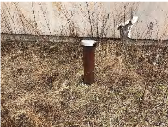
Photo No. 23 IW-1 in good condition
