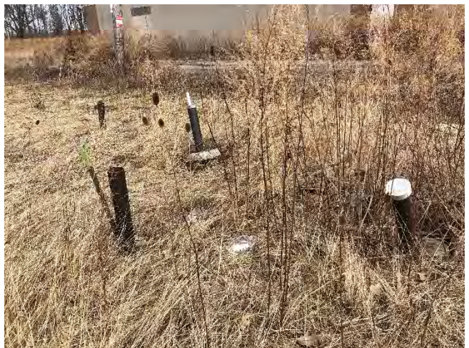
Photo No. 24 Damaged well cluster north of shed
