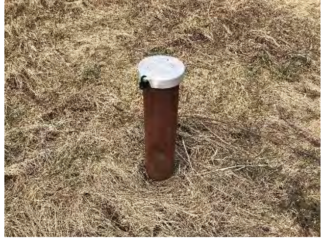
Photo No. 8 IW-8 in good condition
