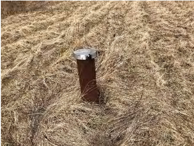
Photo No. 7 IW-12 in good condition
