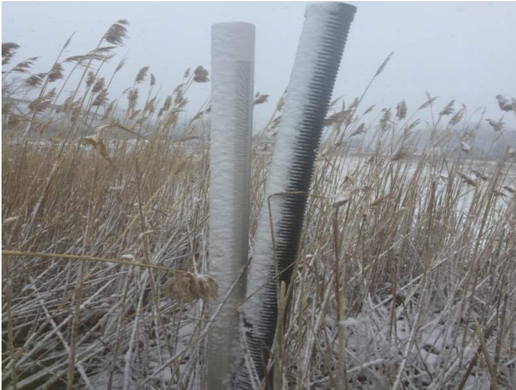
Photo 3c. Nested pair of risers/monitoring well for the product monitoring trench on site.
