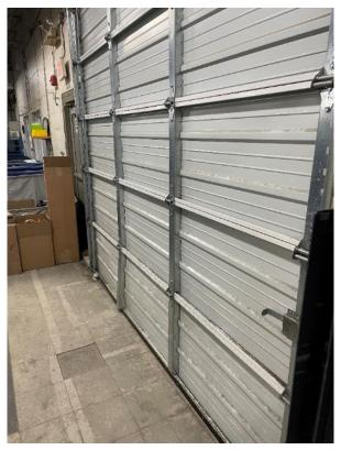
Photo 20 – View of new overhead door on Luther Ave side of the building which provides improved seal.
