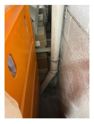
Photo 13 – View of SSDS riser at suction point #8, bollard installation recommended for protection.
