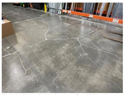
Photo 18 – View of sealed surface cracks in interior concrete floor slab located in main warehouse portion of building.
