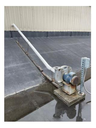
Photo 09 – View of SSDS Fan 1 and pipe supports.
