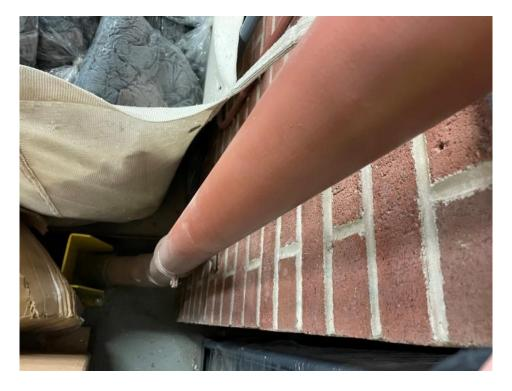
Photo 19 – View of bollard installed at S-11 to protect the suction riser from impact damage.
