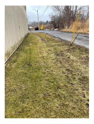
Photo 01 - View of minor soil rutting near western corner of building along Albion Avenue (not on the BCP Site). Recommended to be repaired when weather conditions allow.
