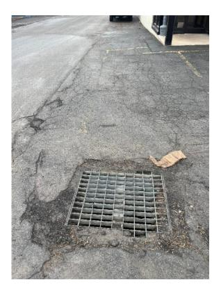
Photo 07 – View of cracked and deteriorated asphalt pavement around stormwater catch basin near Knapp Street and Albion Avenue intersection.
