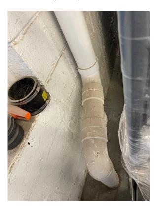
Photo 14 – View of SSDS riser at suction point #14, bollard installation recommended for protection.
