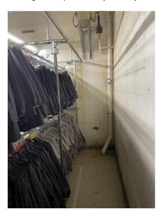
Photo 12 – View of typical SSDS suction point riser and magnehelic gauge.
