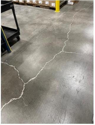
Photo 17 – View of sealed surface cracks in interior concrete floor slab located in main warehouse portion of building.
