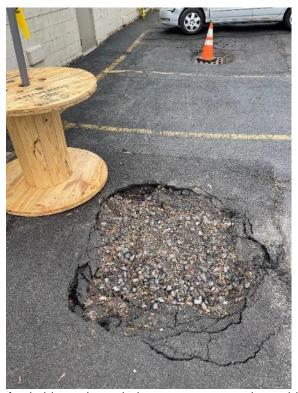
Photo 08 – View of area of subsidence in asphalt pavement on northern side of Site building.
