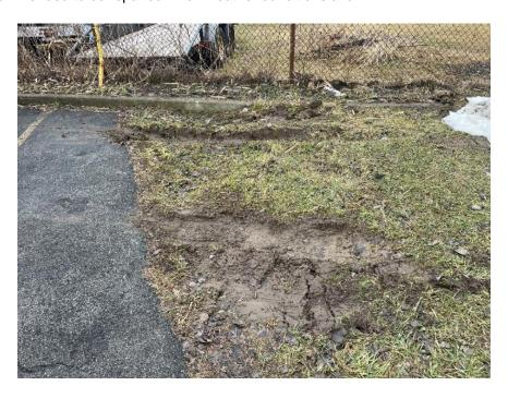
Photo 02 - View of minor soil rutting on the southwest side of the Site near end of Albion Avenue. Recommended to be repaired when weather conditions allow.
