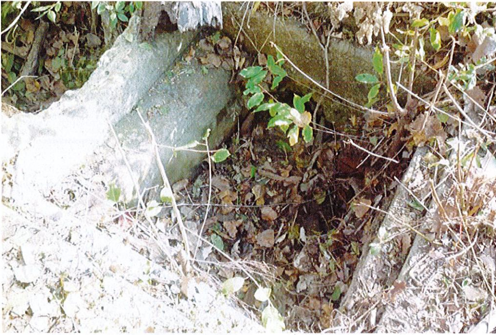
01 Interior of catch basin.jpg
