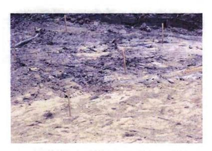
Sand being placed at the bottom of excavation
