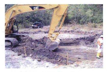
SB-E4 being excavated, top 18 inches removed prior to removing to 4'
