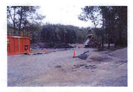
Soil from hot spot locations are staged in lined staging area
