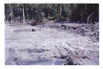
Area 1 showing deeper excavations performed in hot spots
