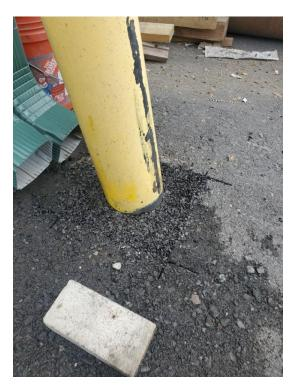
Photograph 20: View of bollard repair with patched asphalt.
