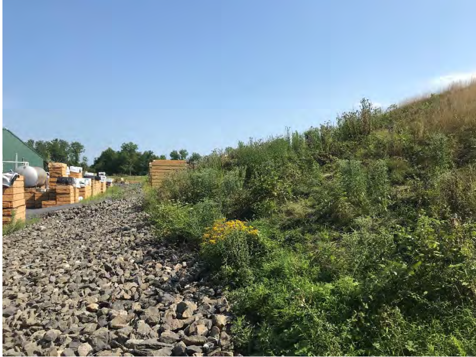
Photograph 13: Grade transition area between treatment process building and storage area in acceptable condition. Looking north.
