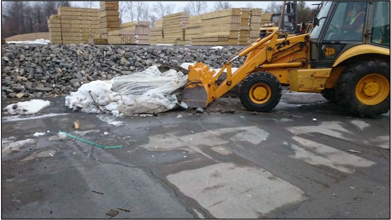
Photograph #6 – Outfeed Deck Soil Disposal
