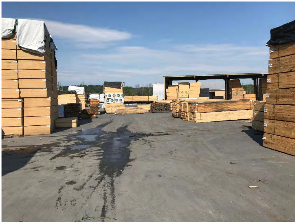
Photograph 12: Southern portion of protective asphalt cover with development of localized depression, but remains in acceptable condition with no penetration. Looking west.
