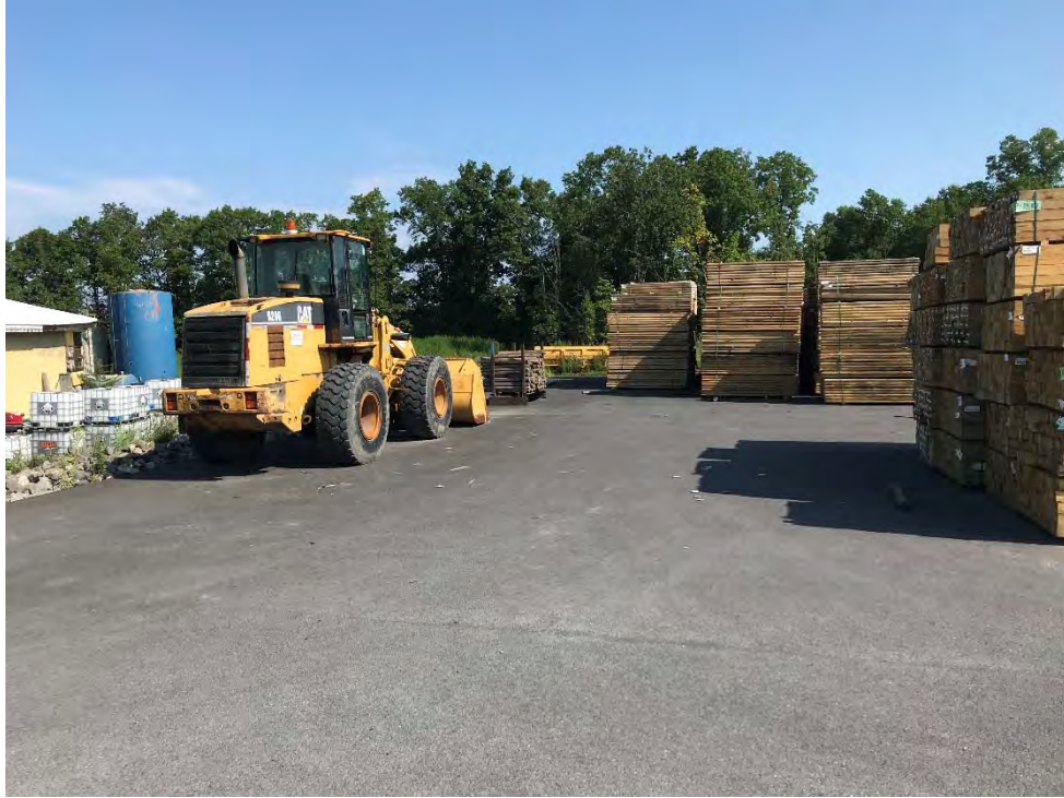
Photograph 11: Northern portion of protective asphalt cover in acceptable conditions. Looking north.
