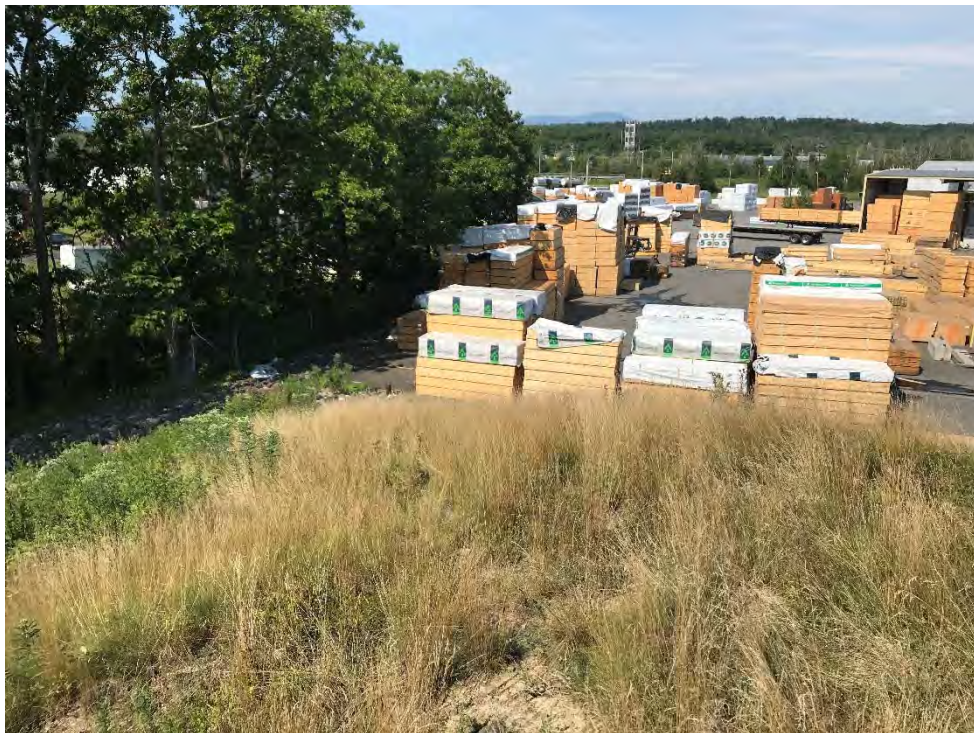
Photograph 4: Southeastern portion of protective asphalt cover and southern abatement berm soil cover in acceptable condition. Looking west.
