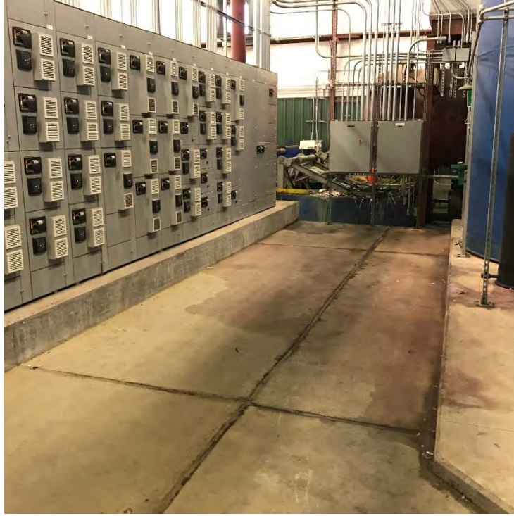
Photograph 19: Representative concrete protective cover in acceptable condition within treatment process building.
