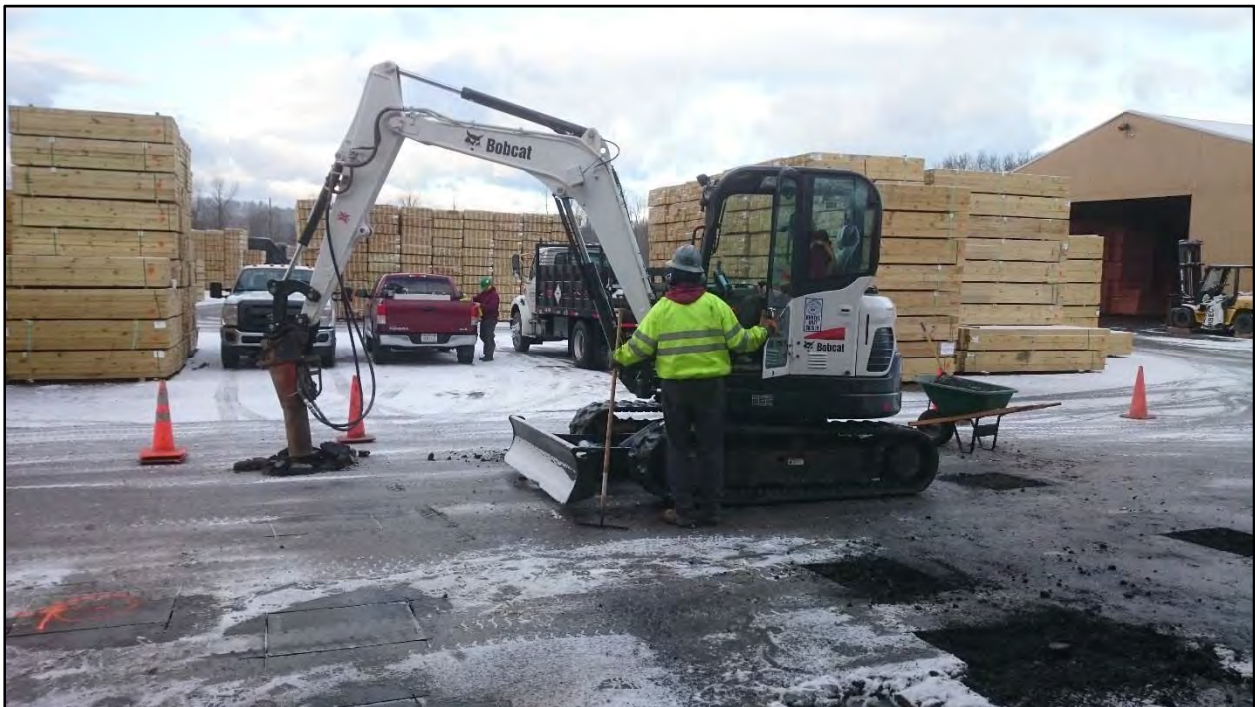
Photograph #2 – Jackhammering and Removal of Asphalt by MCES.
