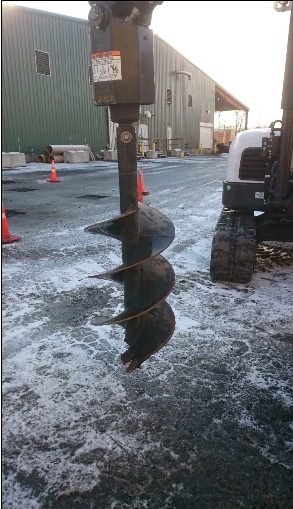
Photograph #3 – Augering & Installation of Feeder Deck Piers by MCES.
