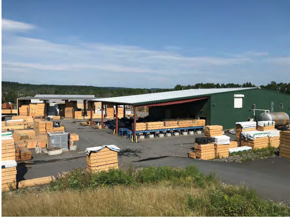
Photograph 3: Overview of eastern portion of protective asphalt cover in acceptable condition. Looking northwest.
