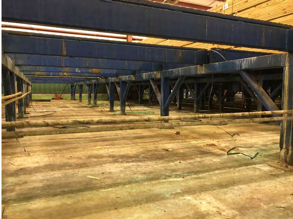
Photograph 18: Representative concrete protective cover in acceptable condition within treatment process building.
