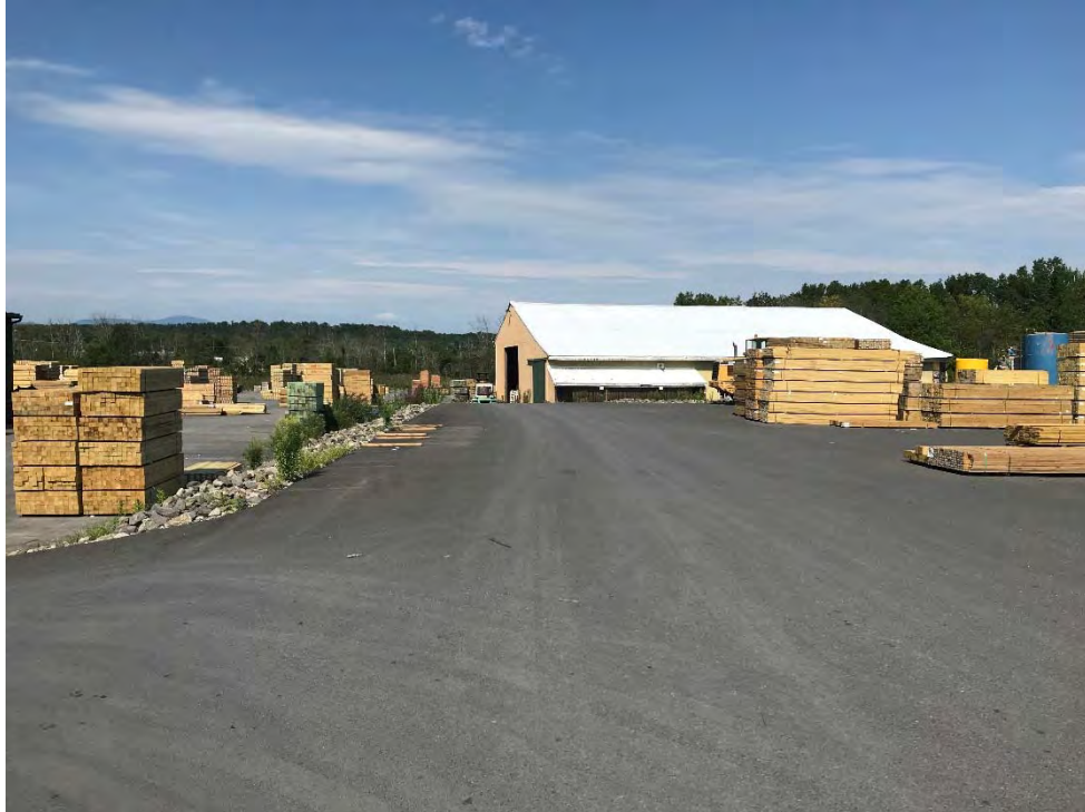
Photograph 10: Northern portion of protective asphalt cover in acceptable conditions. Looking west.
