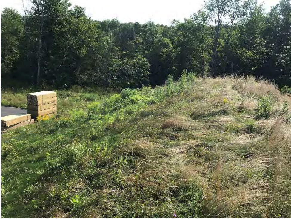
Photograph 5: Southern abatement berm with soil cover in acceptable condition. Looking east.
