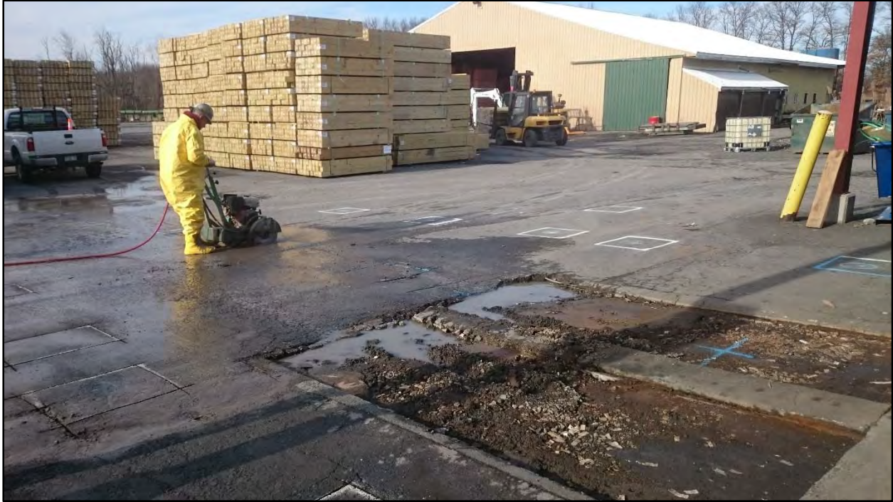
Photograph #1 –Asphalt removal by MC Environmental Services (MCES).
