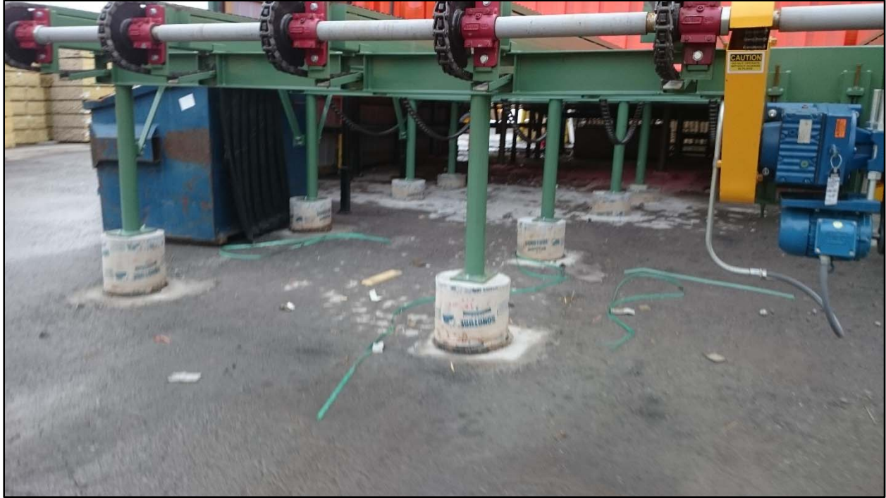
Photograph #4 – Outfeed Deck Piers
