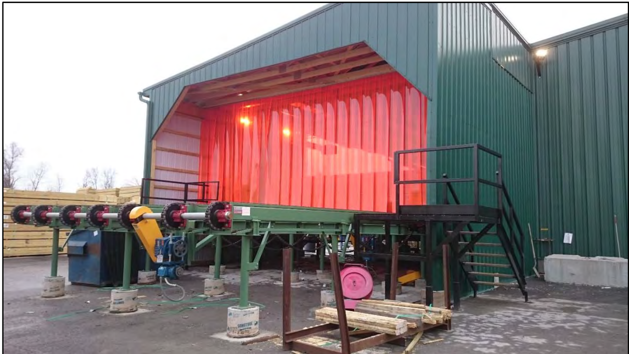
Photograph #5 – Completed Outfeed Deck
