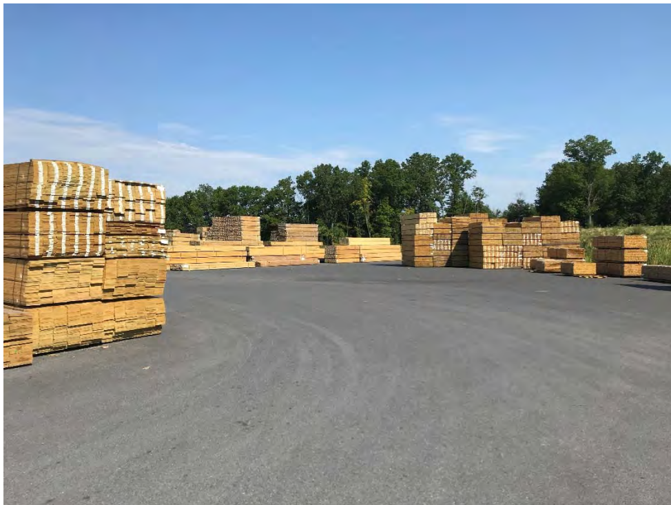
Photograph 8: Northwestern portion of protective asphalt cover in acceptable condition. Looking northwest.
