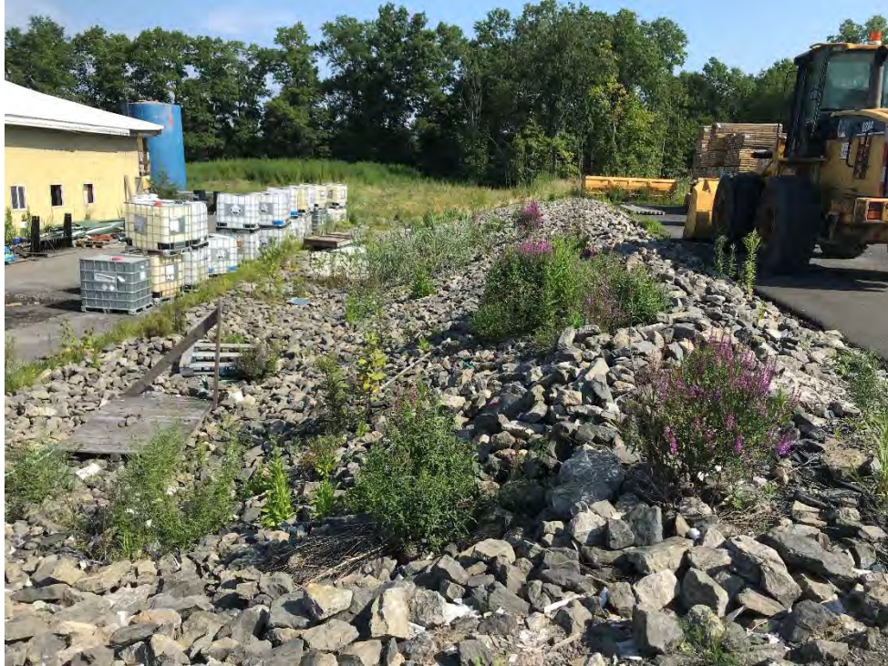
Photograph 14: Northern grade transition area in acceptable conditions. Looking north.
