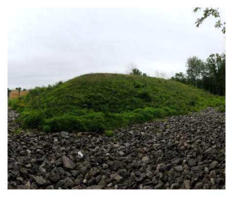
Photograph 6: Abatement berm, facing northeast. Soil cover in acceptable condition.
