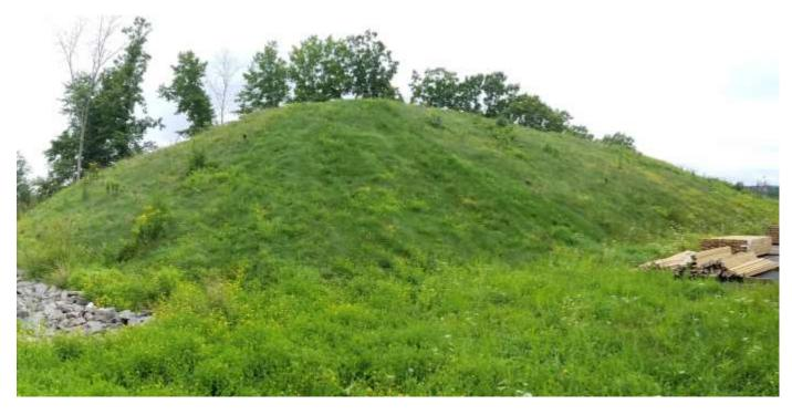
Photograph 5: Abatement berm, facing southwest. Soil cover in acceptable condition.
