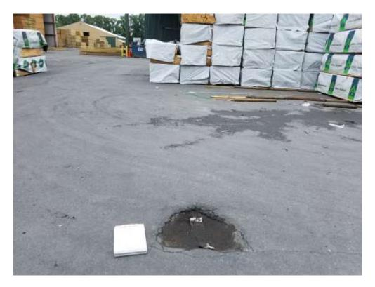
Photograph 1: Depression in asphalt pavement at southwestern portion of Site.
