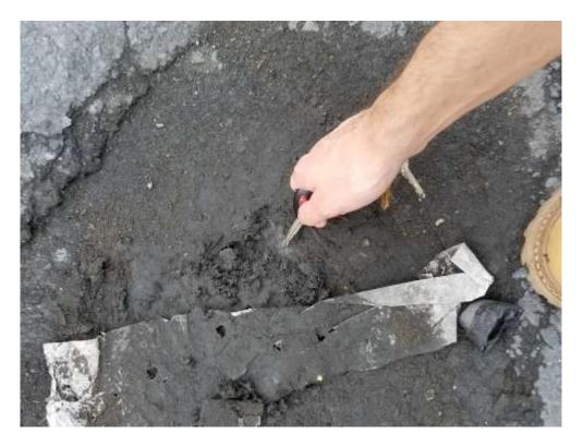
Photograph 2: No penetration observed within the depression of the asphalt pavement.
