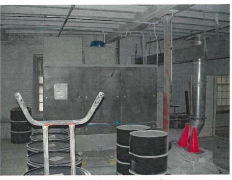
Photo #3: One of the three dust collectors on the 2<sup>nd</sup> Floor of Building 'C'.
