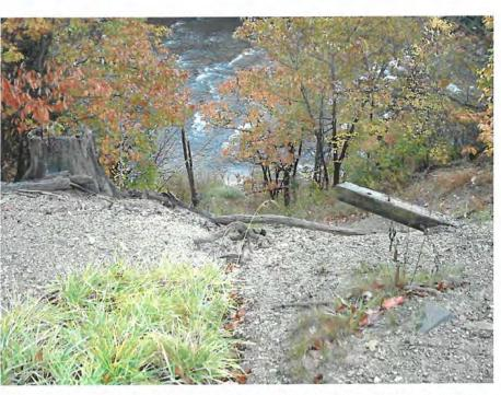
Photo #15: Collapsed slope along the south side of the 'waste pits' area.
