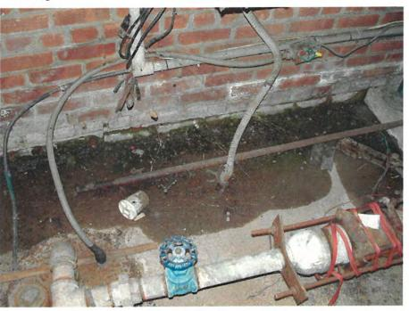
**Photo #8:** Floor of the water pump building, showing hydrocarbon staining on the floor under the previously leaking transformer.
