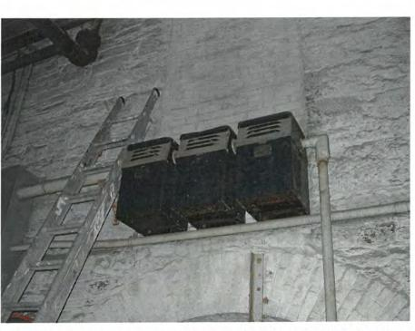
**Photo #9:** The three active transformers in Building 'B', which do not appear to have leaked.
