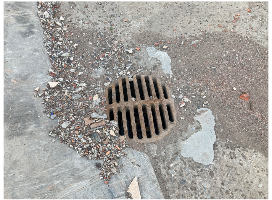
Fig B - Floor Drain
