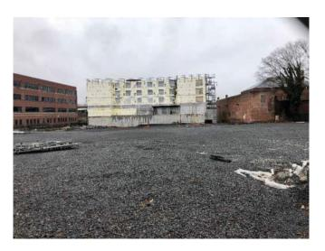
Photo No. 3 West portion of site stabilized with crusher run.
