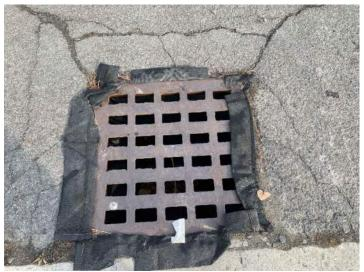
Photo No. 1 View of the site. Photo No. 2 Inlet protection effective.
