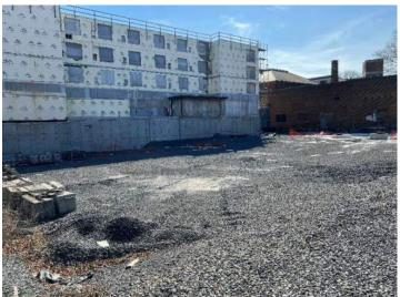
Photo No. 1 Cleanout of silt sack recommended.
