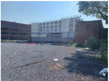
Photo No. 1 Grades stabilized with crushed stone. Looking north.
