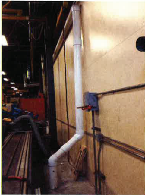
Photograph 7: View looking south at the EEA 4-inch diameter G10P PVC duct and withdrawal location. The system is observed to travel parallel with the east wall in the top of the photograph.
