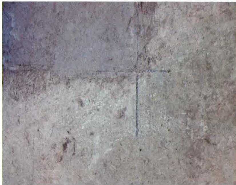
Photograph 6: View of the non-shrinking grout placed in the WEA footprint (top left corner) to the similar grade of the existing concrete slab. Saw-cut locations past the excavation were sealed using the non-shrinking grout.
