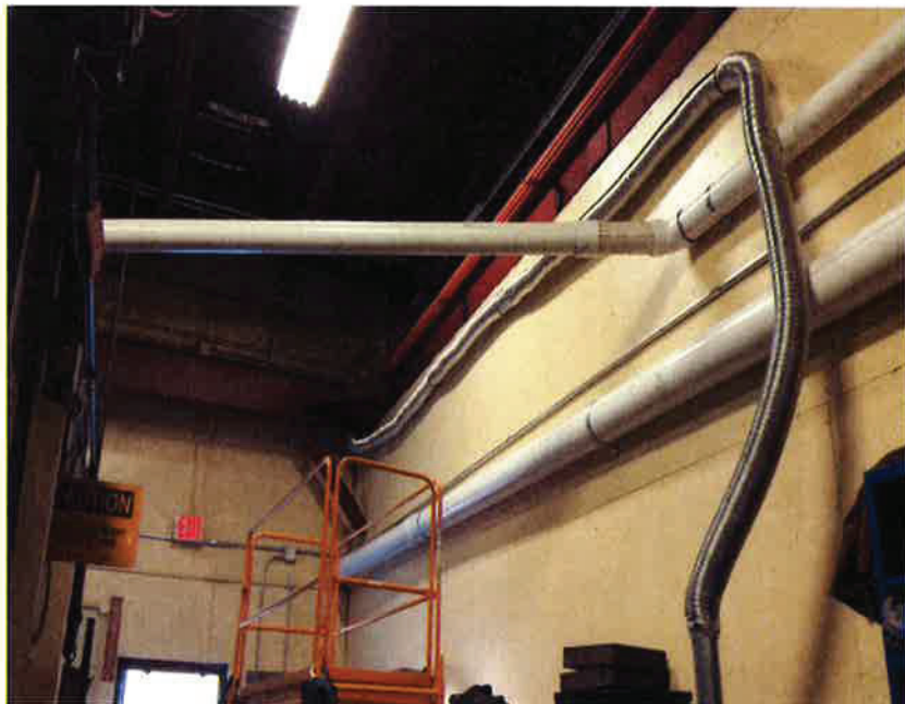
Photograph 10: View of the WEA duct system extending from the left to the right of the photograph, and turning to be parallel with the east wall. Also, the 6-inch diameter duct extends from the right of the photograph to the center to the exterior building wall after exiting the carbon canisters.
