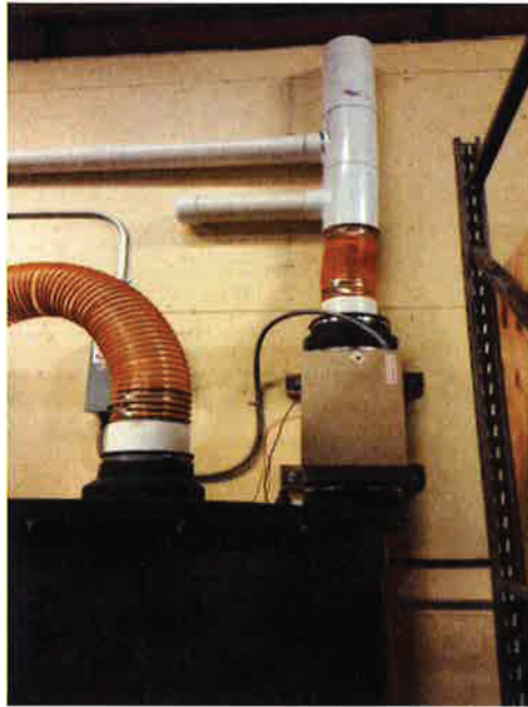
Photograph 11: View looking east at the 4-inch diameter duct from the WEA entering into the 6-inch manifold at the top of the photograph. The bottom tee faces the wall and receives the 4-inch duct (not visible) from the EEA. The bottom tee of the manifold is observed below the 4-inch WEA duct and is capped for future use if needed. The EM-HX 10 Electric Heater is in the center of the photograph and the first G-10P carbon canister is observed in the bottom right.
