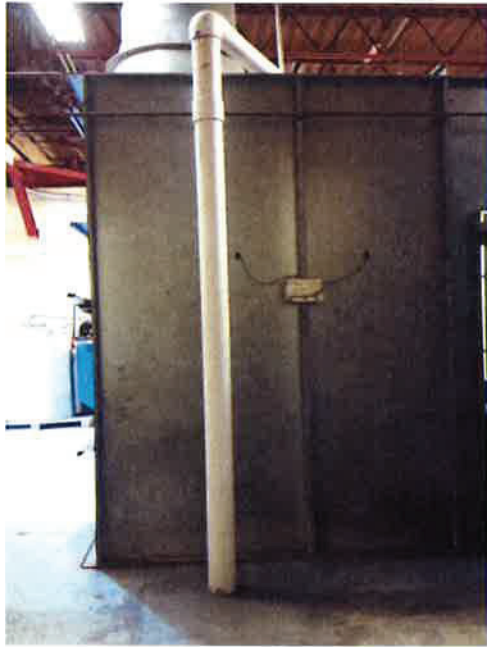
Photograph 9: View looking east at the WEA 4-inch diameter PVC duct exiting the concrete slab. The duct extends from the WEA, into a 90° elbow and horizontally to the southeast over the paint booth.
