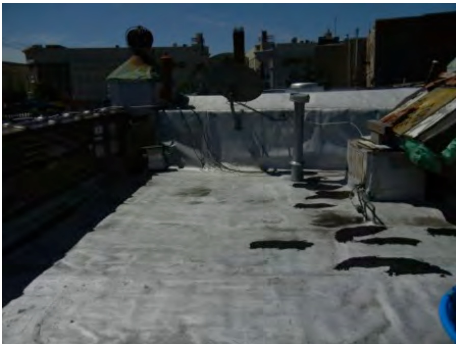
The roofs of the buildings.
