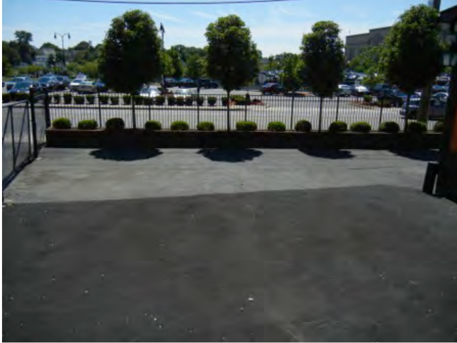
An asphalt parking lot at the property.
