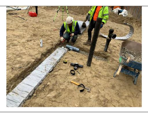
Photo 22: View of SSDS being installed in F3, 4/26/22
