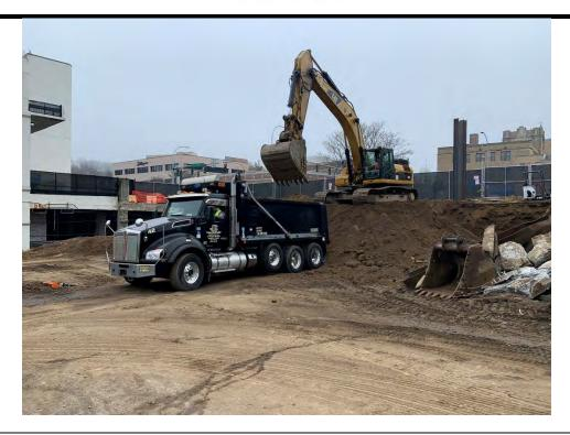
Photo 7: View of soil exporting process beginning on 2/22/22 with the removal of F1-F4 (0-7)
