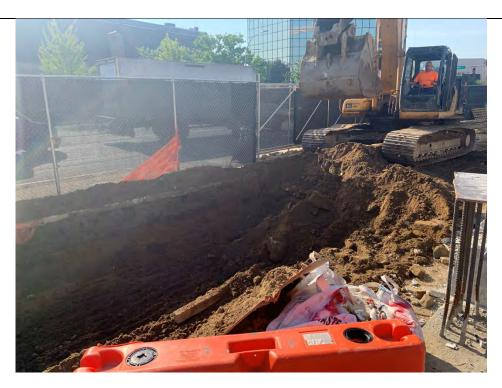
Photo 28: View of excavation to clean end points outside the sheeting line in F3, 7/21/22
