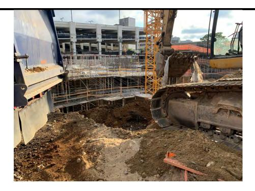
Photo 27: view grid A'3 being exported which represents the last of the native soil inside the SOE, excluding clean fill, 7/12/22
