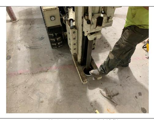
Photo 26: View MW-1 being installed, 7/1/22
