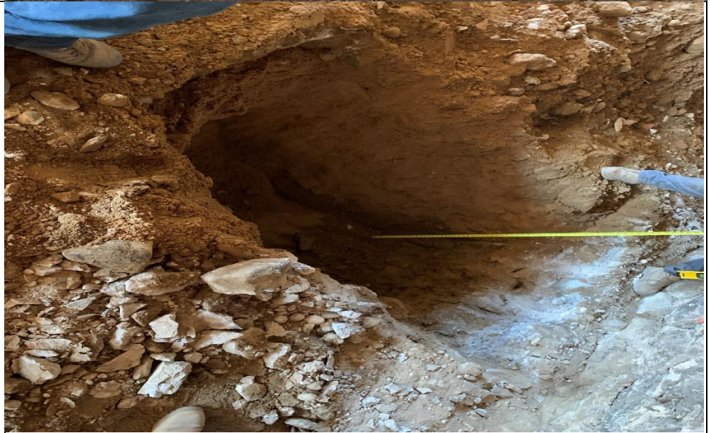
Photo 2 – View of test pit excavation along northern wall on the first floor
