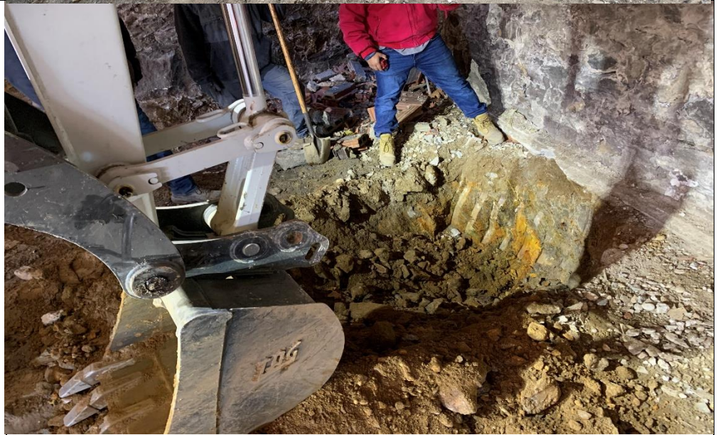
Photo 2 – View of test pit excavation along northern wall on the first floor
