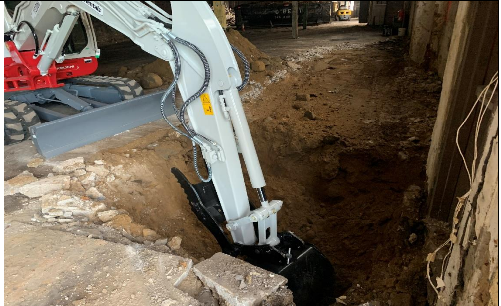
Photo 1 – View of excavation by Southern side wall (1 st floor)
