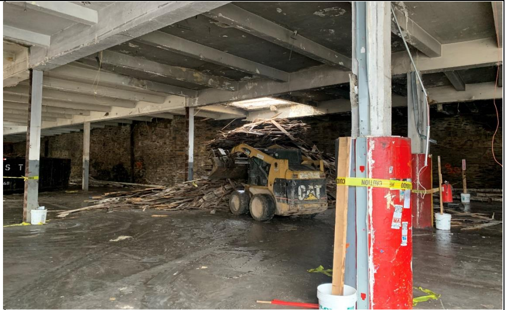
Photo 1 – View of removed wood stockpiling (non scope)
