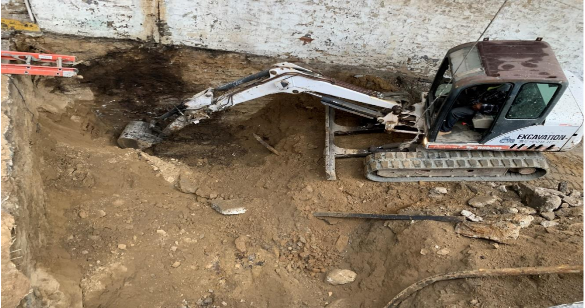
Photo 1 – Excavation of stained soil where the UST was located
