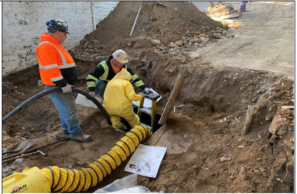
Photo 3 – View of pumping of UST and clean up with absorbent pads
