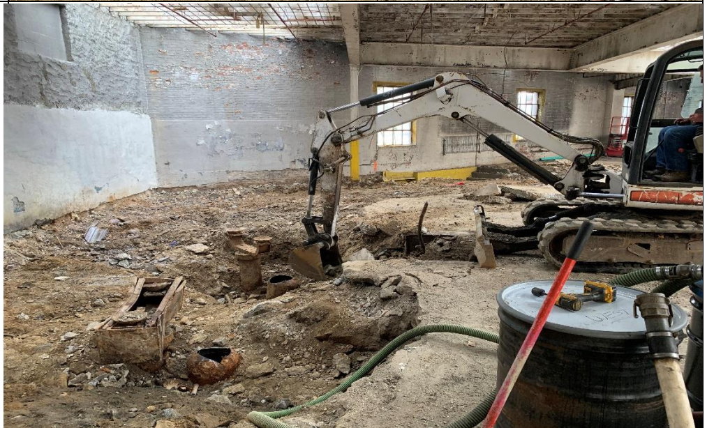
Photo 2 – View of excavation around Eastern most piston
