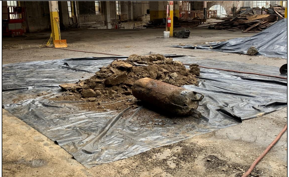
Photo 1 – View of removed Hydraulic fluid tank along with stockpiled soils
