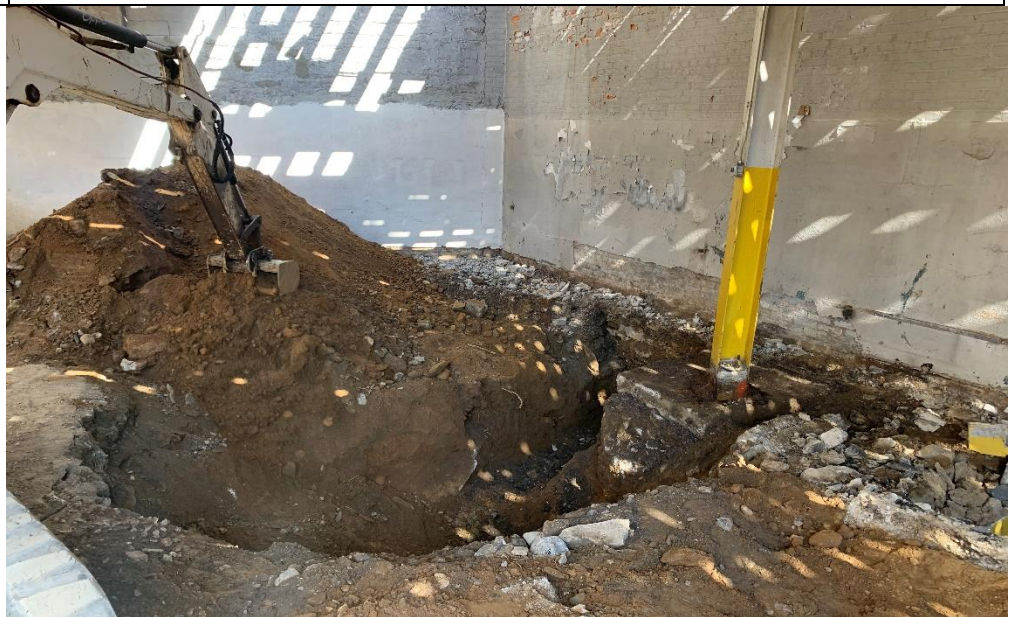
Photo 2 – Excavation around support beam near NE staircase (5-6ft deep)
